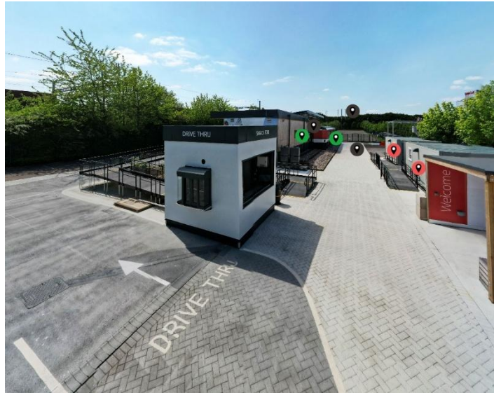
Figure 2 - East to West View across the existing site 3
