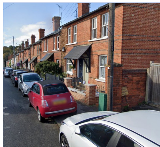
Image 1A – The other slate-roofed porches on Brook Street demonstrating the same style.
