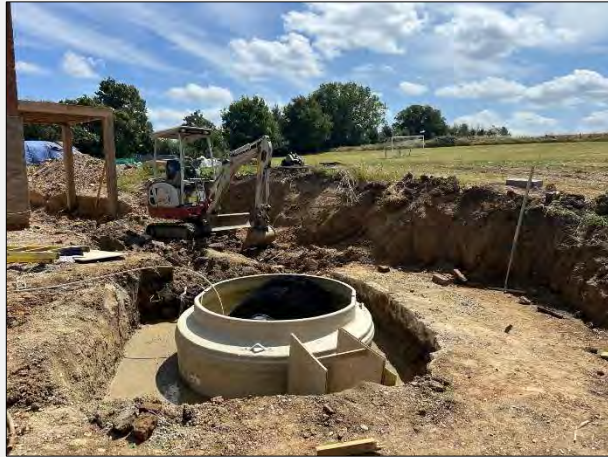
Plate 5: Current construction involving septic tank
