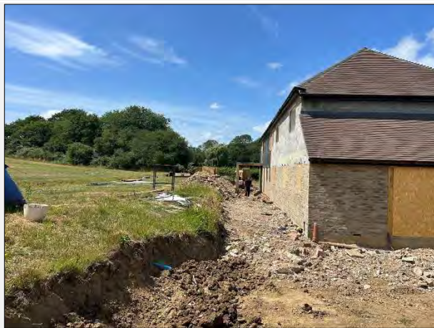
Plate 7: General site view
