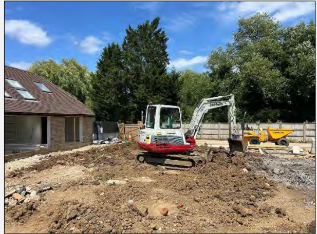
Plate 6: Current construction on site
