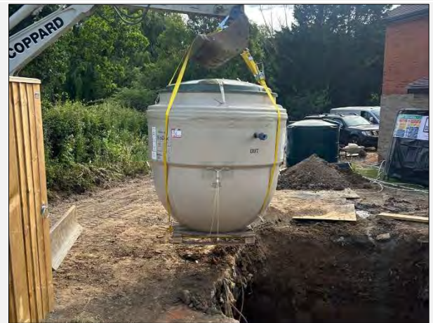
Plate 8: Current construction underway
