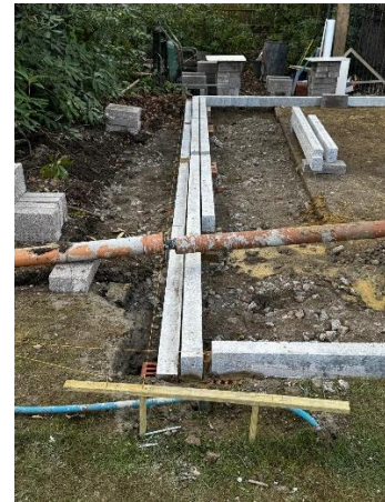
Ground beams on pads
