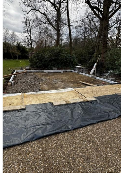
Pad and beam construction
