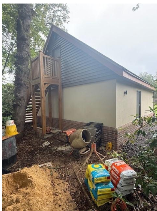
Staircase built off concrete slab
