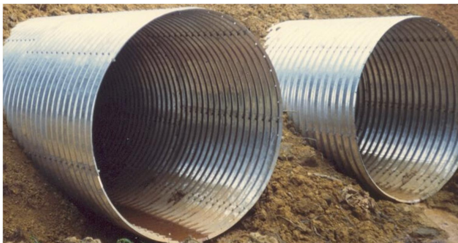
Figure 4-2: Typical Corrugated Storm Drain
