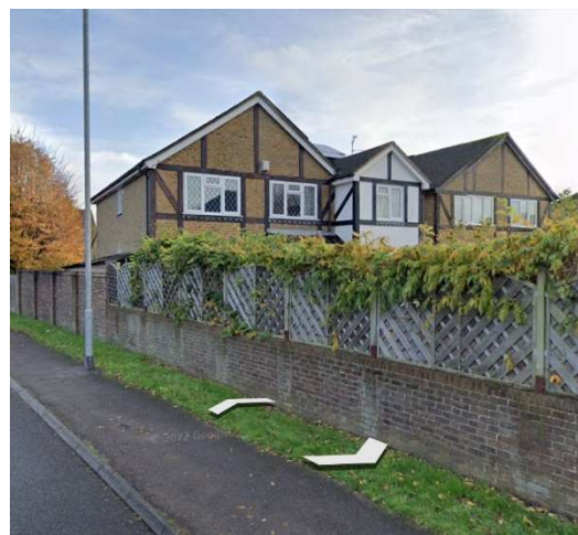
Front Elevation of 8 Wield Court – As seen from the public highway
