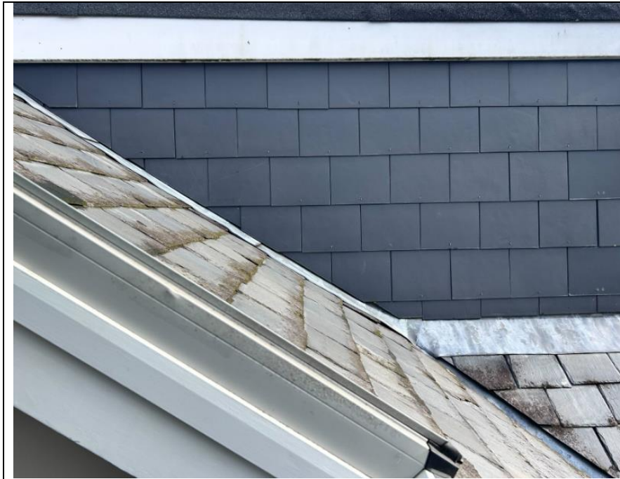
Figure 5: Neighbouring dormer facing east. (Good condition tiles, hanging tiles and flat roof)
