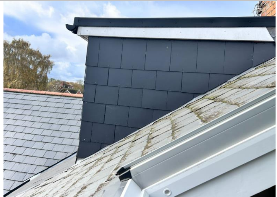
Figure 6: Neighbouring dormer facing west. (Good condition tiles, hanging tiles and flat roof)
