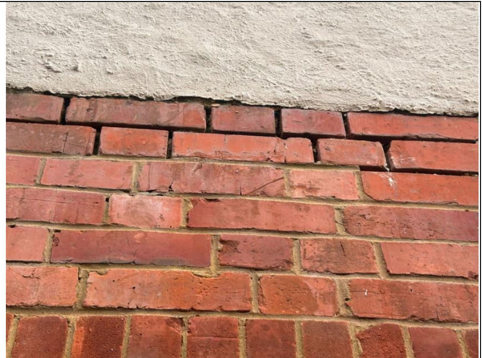
Figure 8: Mortar gaps on the western face.
