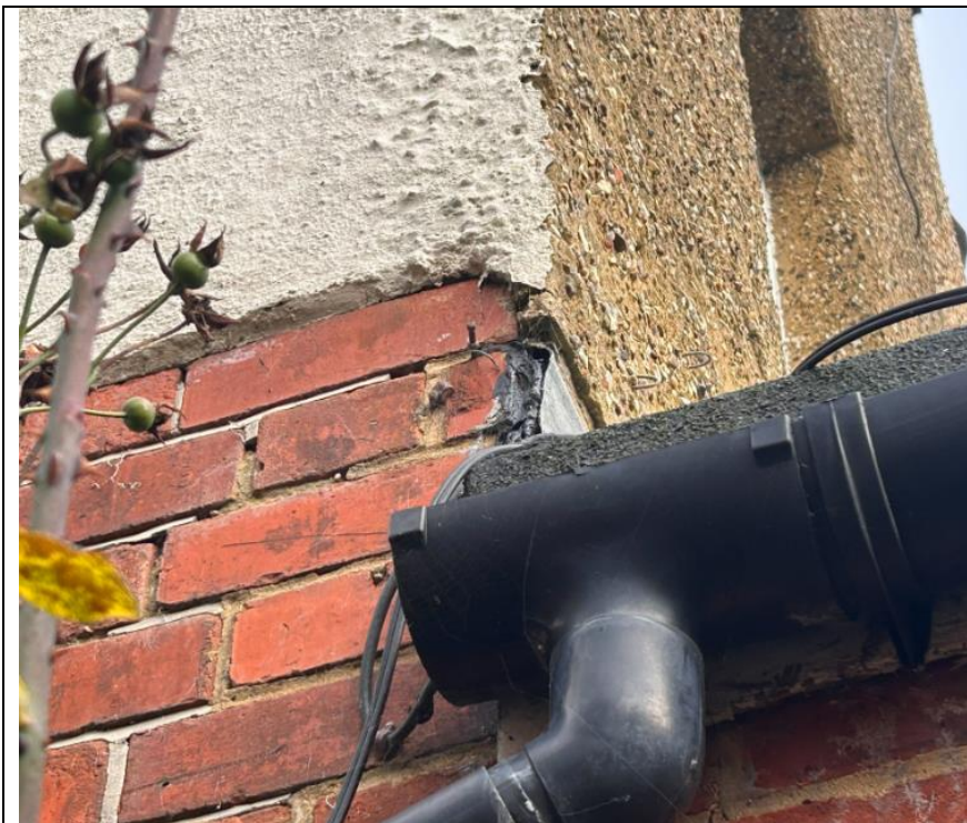
Figure 9: Sealed lead flashing on the western face
