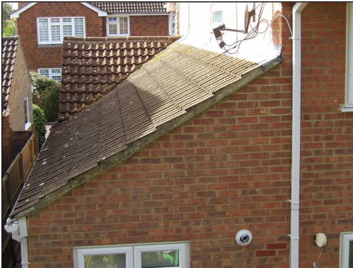
Figure 11. Sealed soffits and fascias around home office/utility. 8 Barholm Close, Lower Earley. 22.10.24
