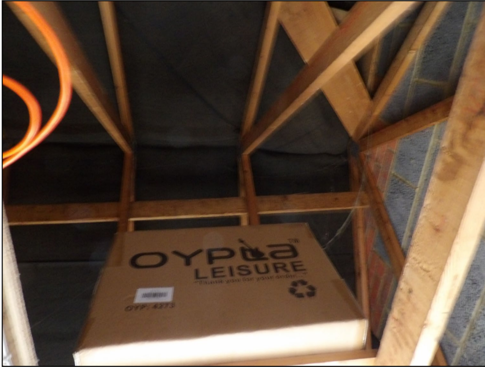
Figure 14. Example of bitumen lining in pitched roof over garage. 8 Barholm Close, Lower Earley. 22.10.24
