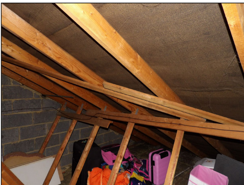
Figure 13. Example bitumen lining in loft. 8 Barholm Close, Lower Earley. 22.10.24
