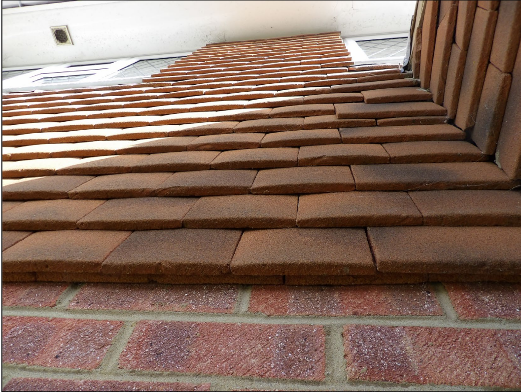
Figure 7. Example well fitted hanging tiles. 8 Barholm Close, Lower Earley. 22.10.24
