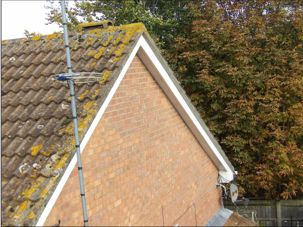
Figure 5. Example sealed verges. 8 Barholm Close, Lower Earley. 22.10.24
