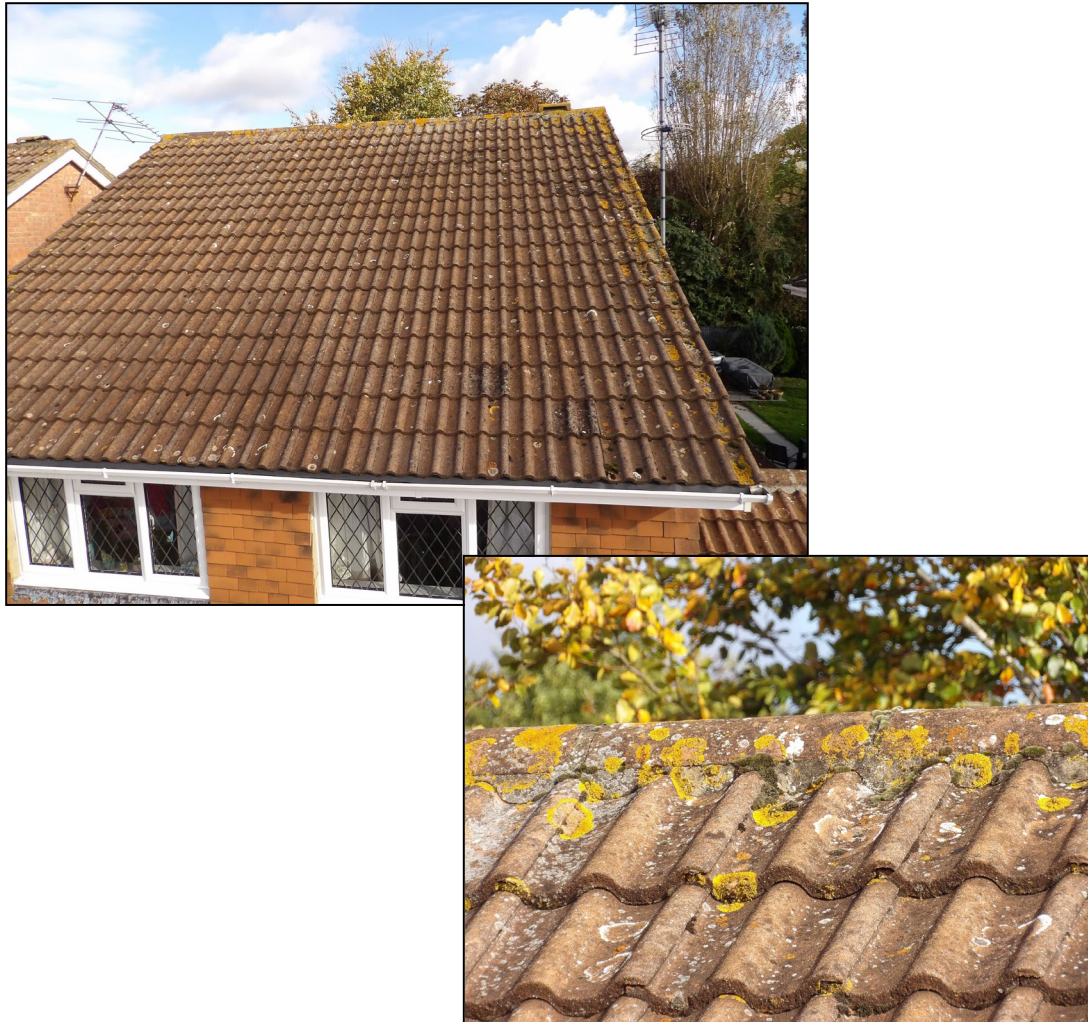
Figure 4. Tightly fitted roof and ridge tiles. 8 Barholm Close, Lower Earley. 22.10.24
