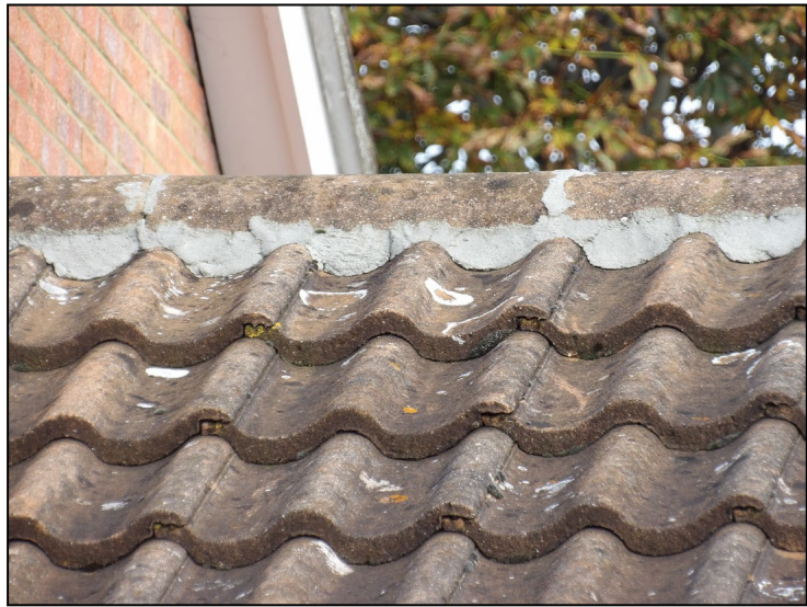
Figure 10. Roof tiles/verges and sealed lead flashing of rear home office/utility. 8 Barholm Close, Lower Earley. 22.10.24
