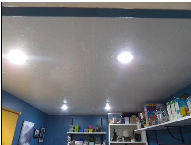
Figure 15. Boarded ceiling of home office/utility. 8 Barholm Close, Lower Earley. 22.10.24
