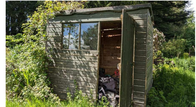
Eastern elevation of B3.
