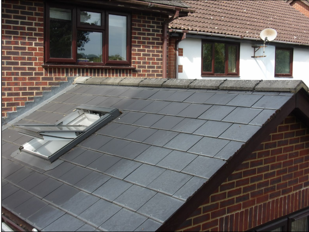
Figure 9. Tightly fitted roof and ridge tiles/Velux window on rear extension. 8 Hunters Way, Spencers Wood, 28.08.24
