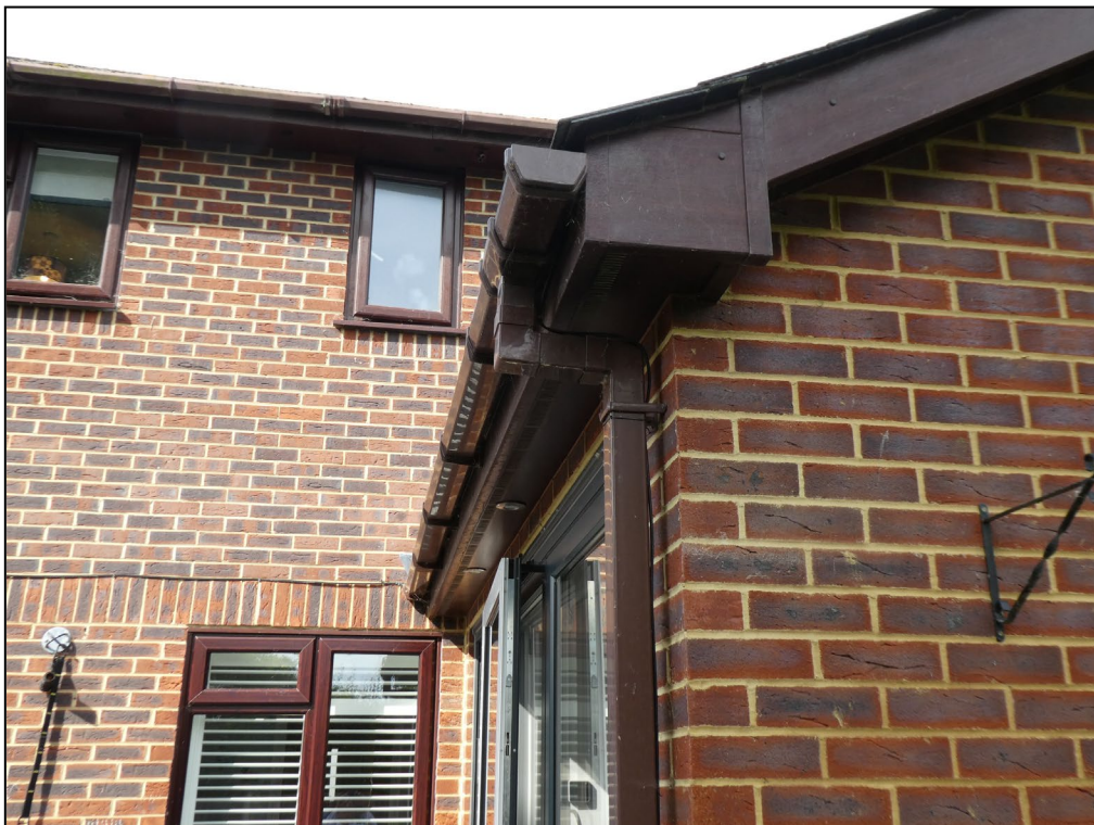
Figure 10. Sealed soffits and fascias on rear extension. 8 Hunters Way, Spencers Wood, 28.08.24
