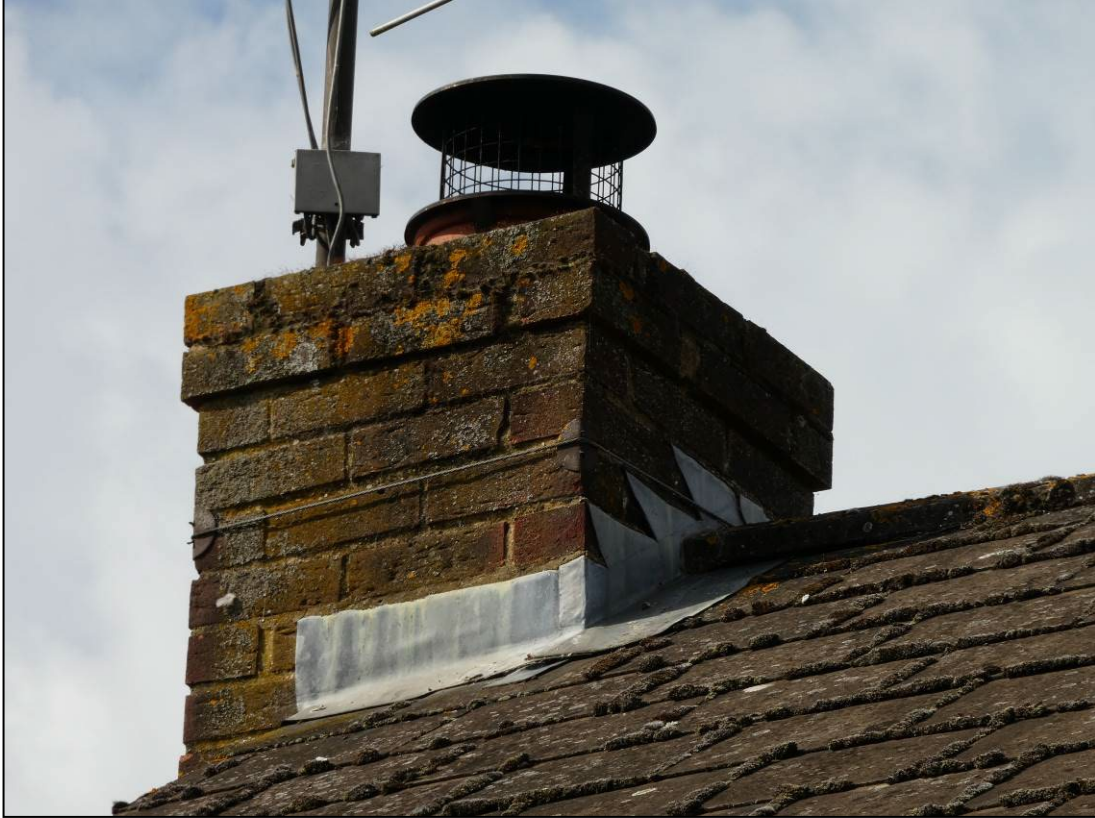
Figure 7. Lead flashing around the chimney. 8 Hunters Way, Spencers Wood, 28.08.24
