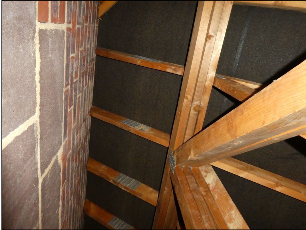
Figure 16. Bitumen lining in garage loft space. 8 Hunters Way, Spencers Wood, 28.08.24
