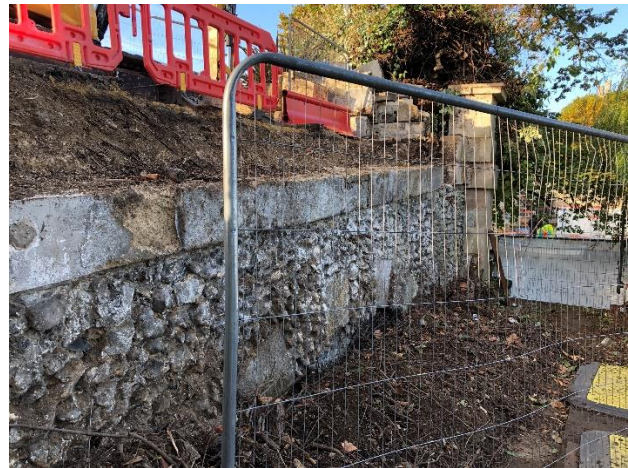
Photo 2: View looking North-West - Exposed flint face retaining wall
