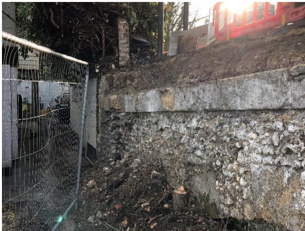
Photo 1: View looking South-East - Exposed flint face retaining wall
