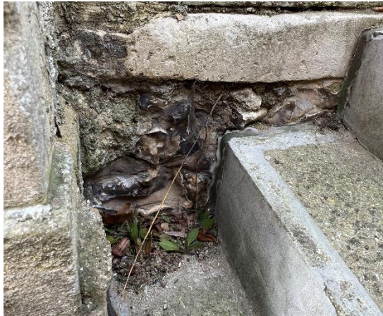
Figure 4 - Flint possibly dating to the 12th century bridge, identified on the south eastern elevation of Henley Bridge.
