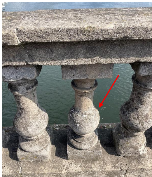
Figure 7 - Balustrade on Henley Bridge's northern elevation. The baluster identified with a red arrow is believed to be from the 1953 or 1981 (Appendix A), whilst the baluster on the right is believed to predate this.
