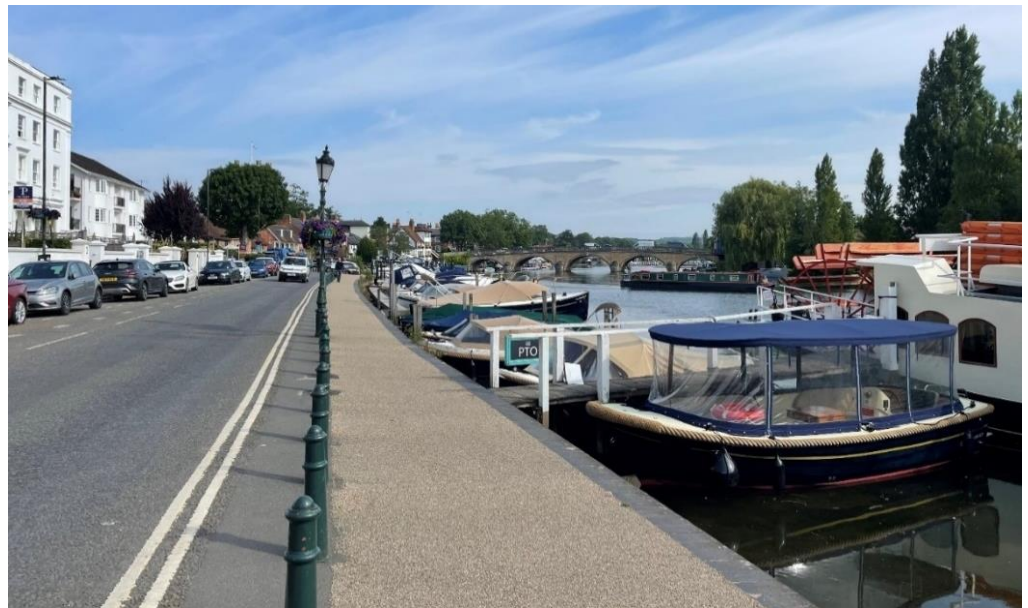
Figure 10 - View of Henley Bridge looking north from an identified important view from Thameside
