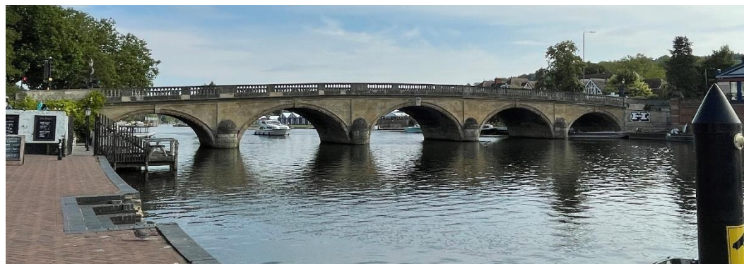
Figure 5- Henley Bridge, Southern elevation
