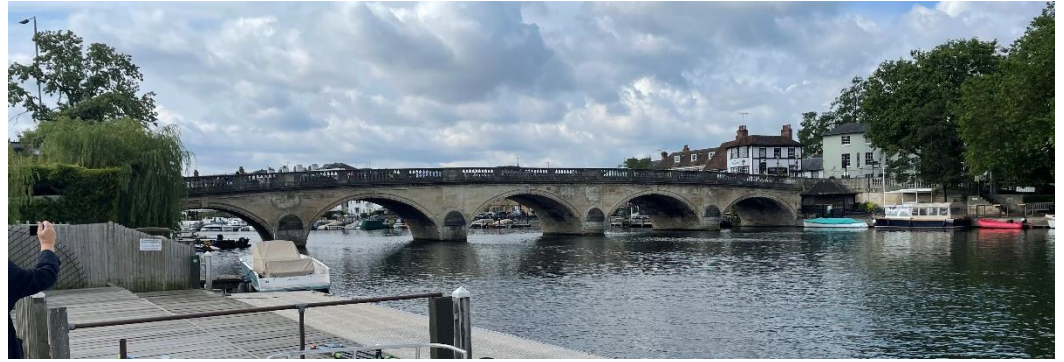
Figure 6 - Henley Bridge, Northern elevation
