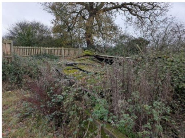
Image 9: Collapsed shed with bramble scrub.
