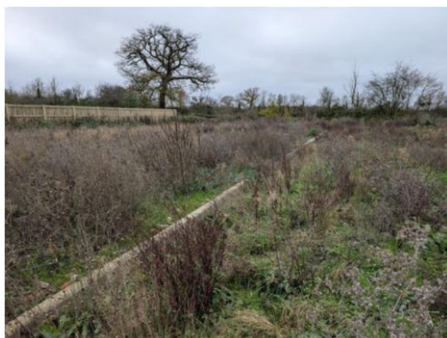
Image 12: Concrete foundation running along the middle of the ruderal vegetation.
