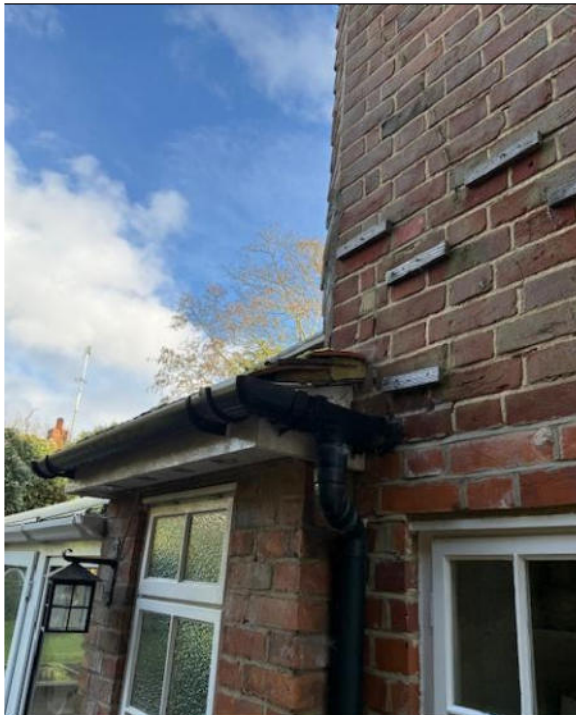
Photograph 13: Rear gutters and soffits.
