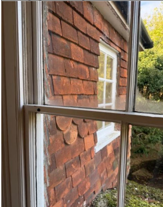
Photograph 7: Hanging wall tiles.
