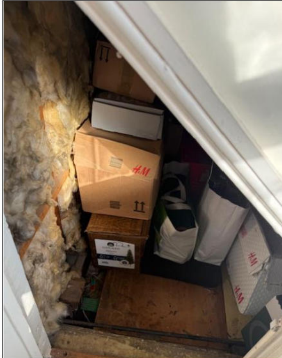
Photograph 1: Eaves space used for storage.
