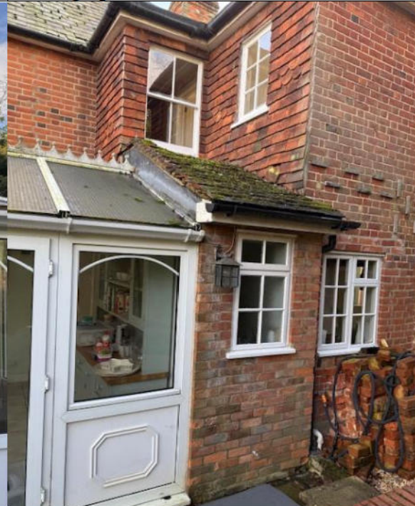
Photograph 12: Rear elevation hanging wall tiles.
