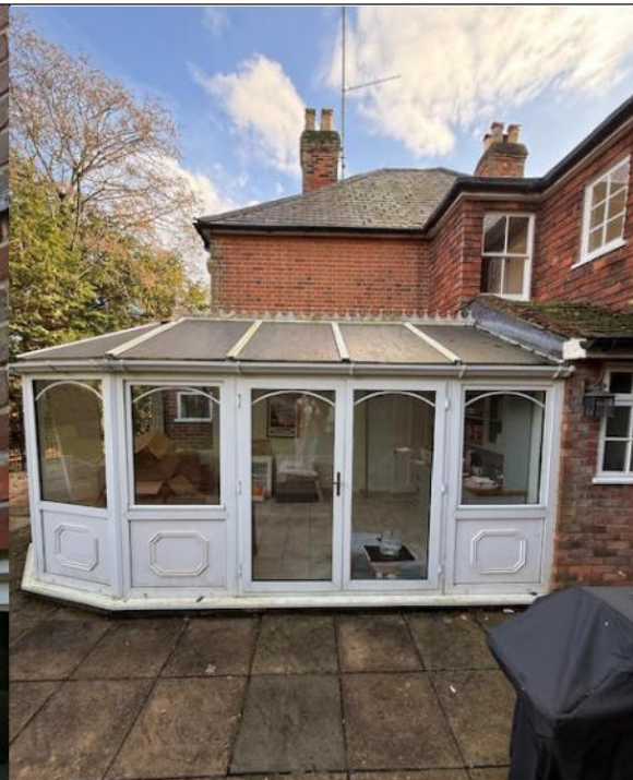
Photograph 14: Conservatory- rear elevation.
