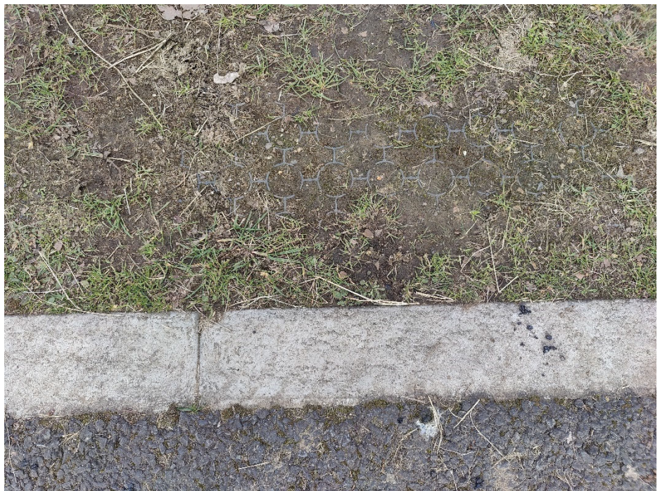
Close up photo taken on the 18 th March 2025 of area adjacent to access where BodPave is installed. Bodpave is partially visible in some areas but it has generally been covered by grass.
