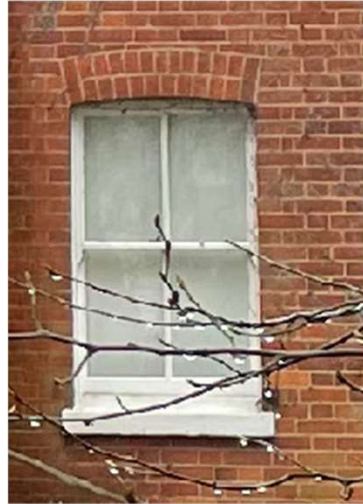
Stone Window Sills / Brick Lintels
