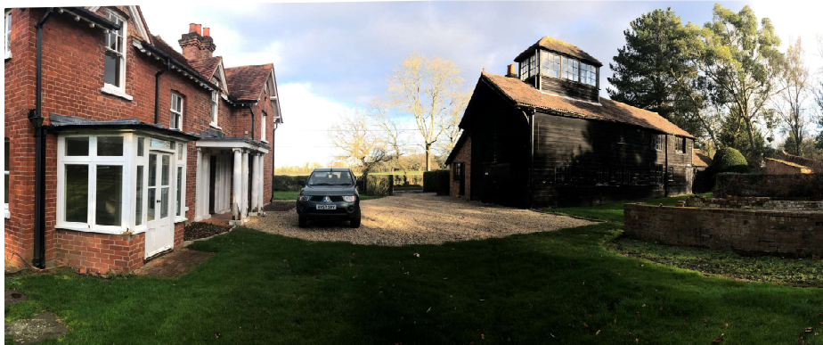
Existing View From South
