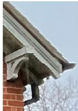
Roof Facias & Eaves
