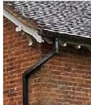
Cast Iron Rain Water Pips
