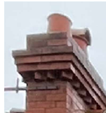
Red Brick Chimneys / Terracotta Flues
