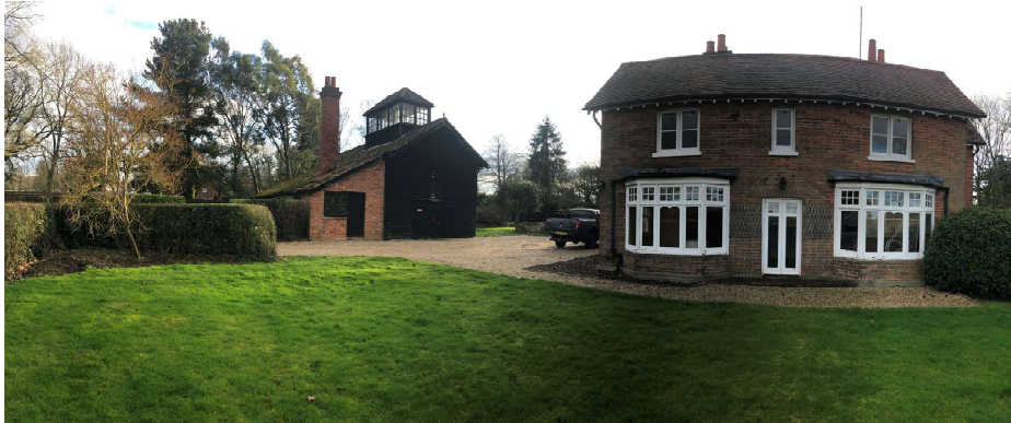
Existing View From North East
