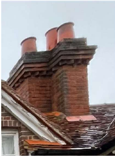
Tiled Roofs / Brick Chimneys / Flues
