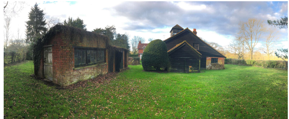
Existing View From South East
