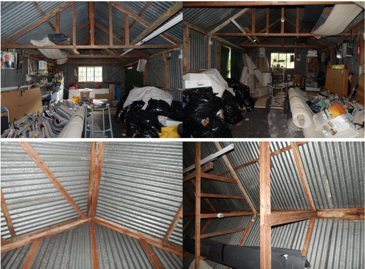
Internal view of B2
