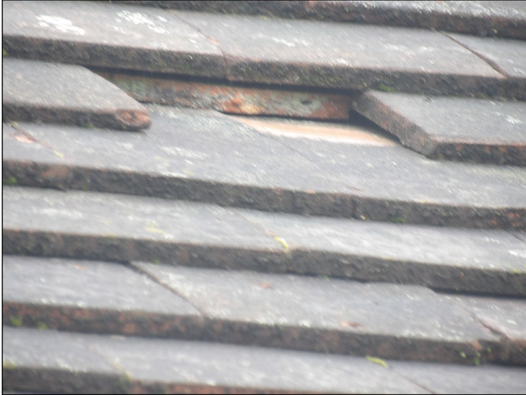
Figure 5. Example of broken tile with stub in situ. 195 Victoria Road, Wargrave. 15.04.25
