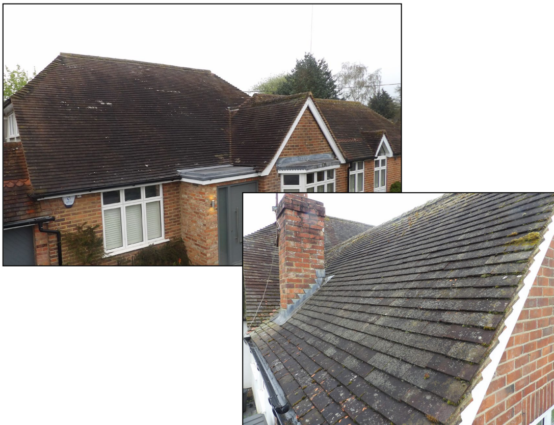
Figure 4. Multi pitched roof and well fitted roof tiles. 195 Victoria Road, Wargrave. 15.04.25
