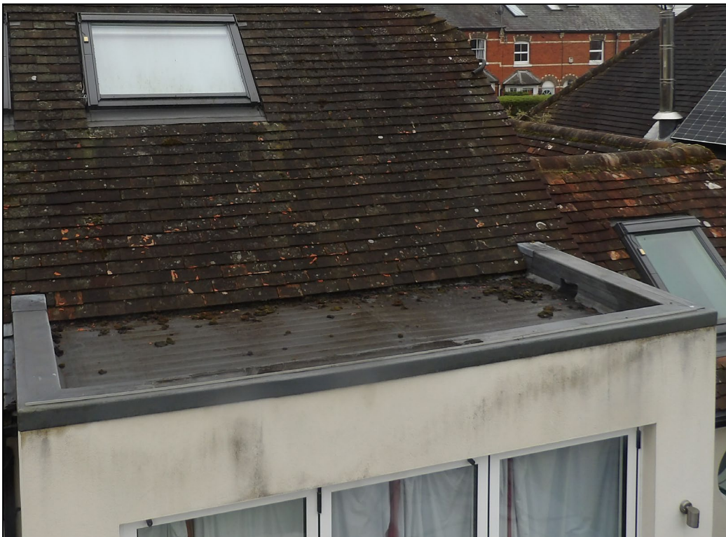
Figure 12. Example sealed lead flashing on extension. 195 Victoria Road, Wargrave. 15.04.25
