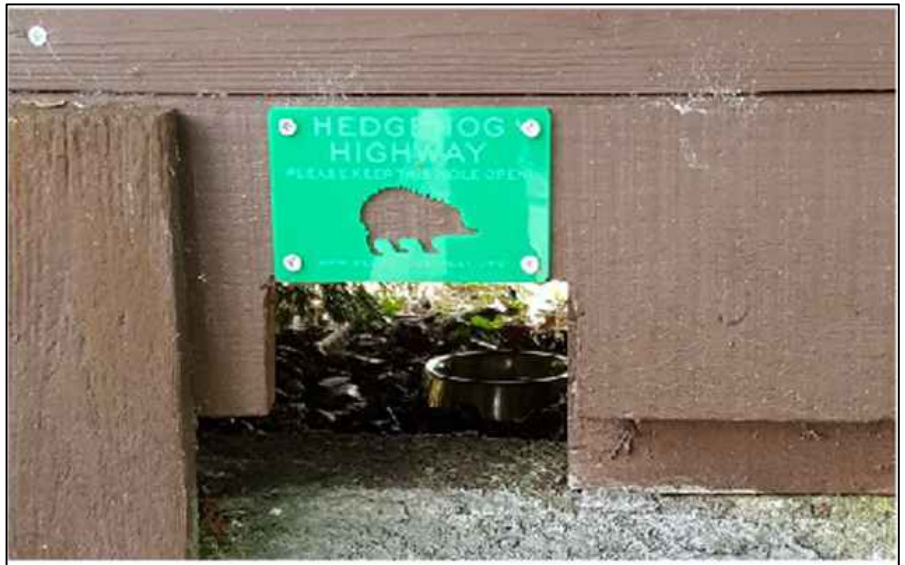
IMAGE ABOVE OF HEDGHOG HIGHWAY, 13X13CM GAP IN FENCE WITH ACCOMPANYING SIGN TO PREVENT ACCIDENTAL BLOCKAGE
