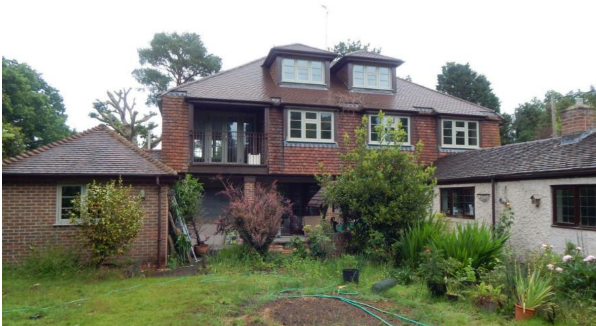
Image 4 – Rear South facing elevation of the property offering further vertical hanging tiles where a single Pipistrelle bats was observed during the assessment
