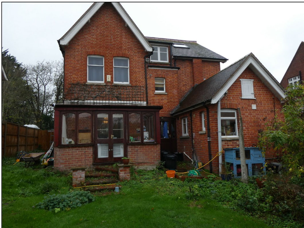
Figure 4. Rear view of property. Hillside House, Spencers Wood. 14.11.25
