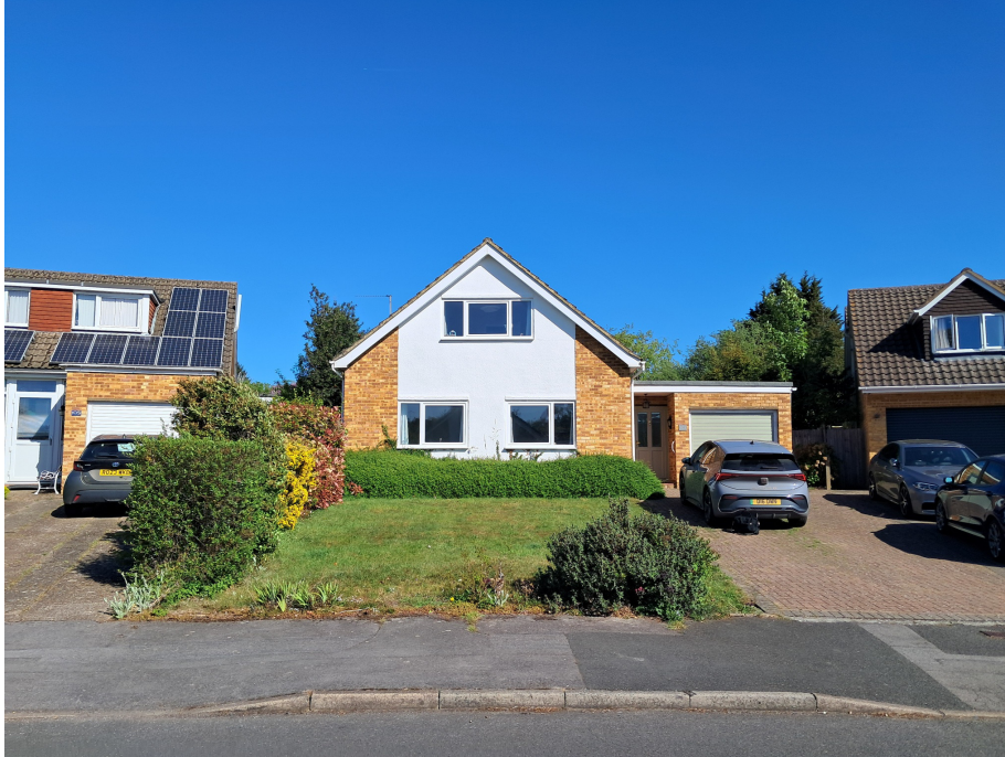
Front Elevation – general view
