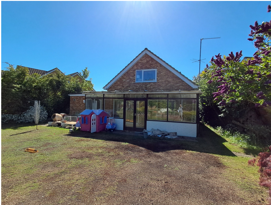
Rear Elevation – general view
