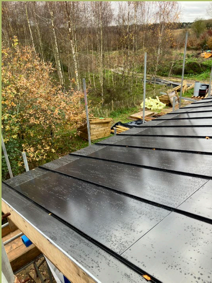
'Roofit' integrated solar at Hawkes project Shurlock Row Barns, a low energy barn conversion near the site.
