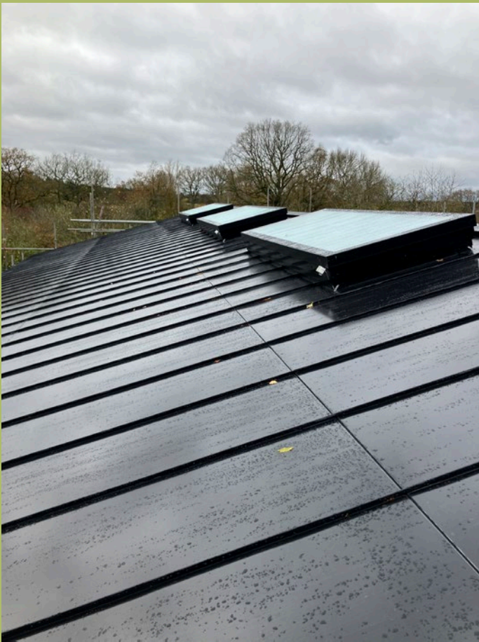
'Roofit' integrated solar at Hawkes project Shurlock Row Barns, a low energy barn conversion near the site.
