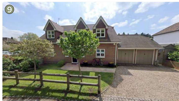
Hamilton House, Hayes Lanes, Barkham Hill [Image Source: Google Street View]
