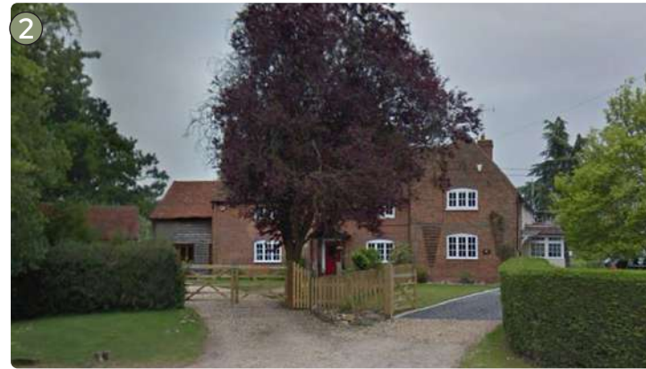
Church Cottages, Church Lane, Old Barkham [Image Source: Google Street View]
