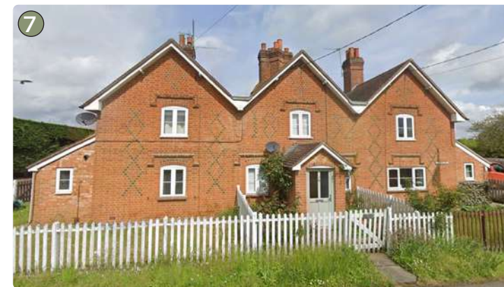
Coppid Hill Cottages, Barkham Road, Barkham Hill [Image Source: Google Street View]
