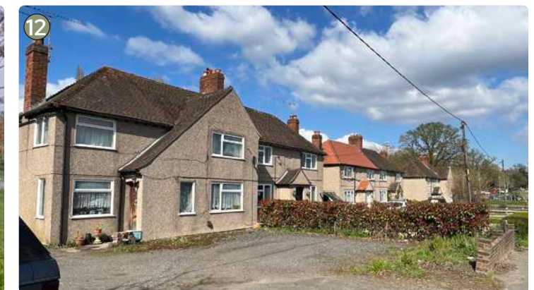
Bridge Cottages, Barkham Road [Image Source: Hawkes Architecture]
