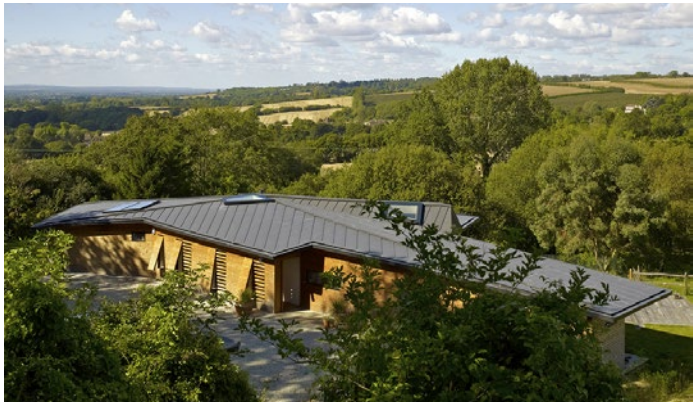
Example of shallow pitched zinc roofing on a contemporary dwelling
