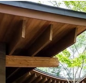
LIGHT TIMBER BATTENS
