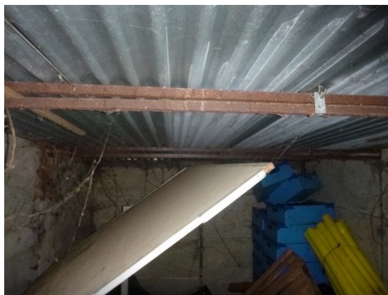
Unlined roof, no crevice opportunities (B4).
