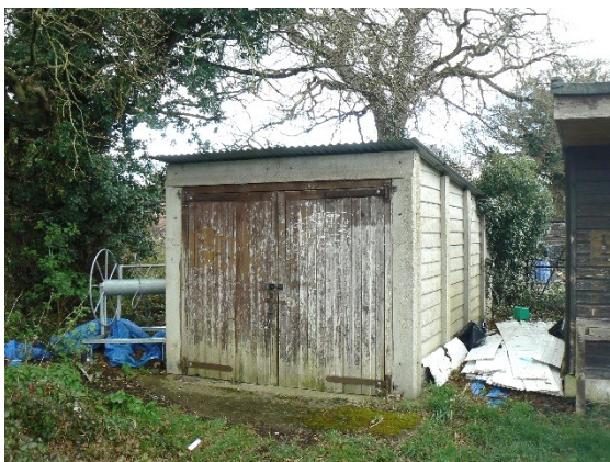
Prefab structure with corrugated roof (B4).
