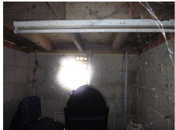
Heavily cobwebbed, sterling board lined, no crevice opportunities (B3).
