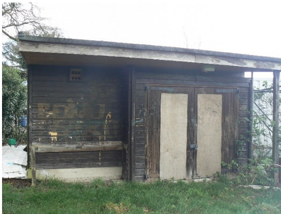
Blockwork timber clad structure with access gaps above doors (B3).
