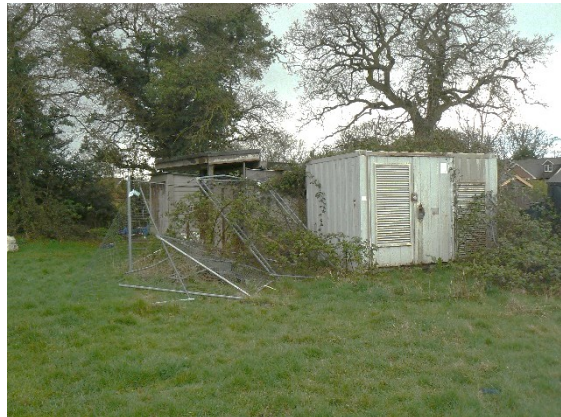
24. Storage structures in western corner (u1b5).
