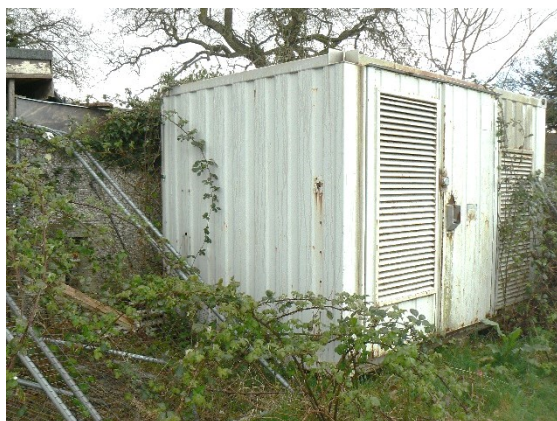
Small metal storage structure with vented/louvred doors (B2).
