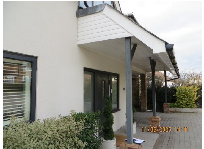
Front roof overhang.
