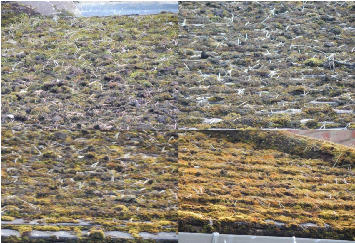
Image 5 – Rear North facing roof coverings which offer a moderate covering from moss which may obstruct visibility of any suitable gaps of value to bats throughout
