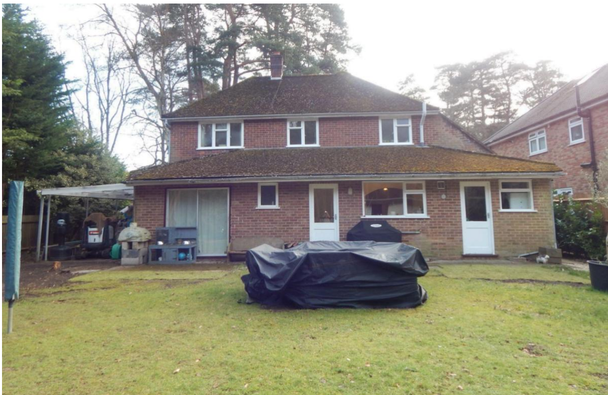
Image 4 – North facing elevation of the property
