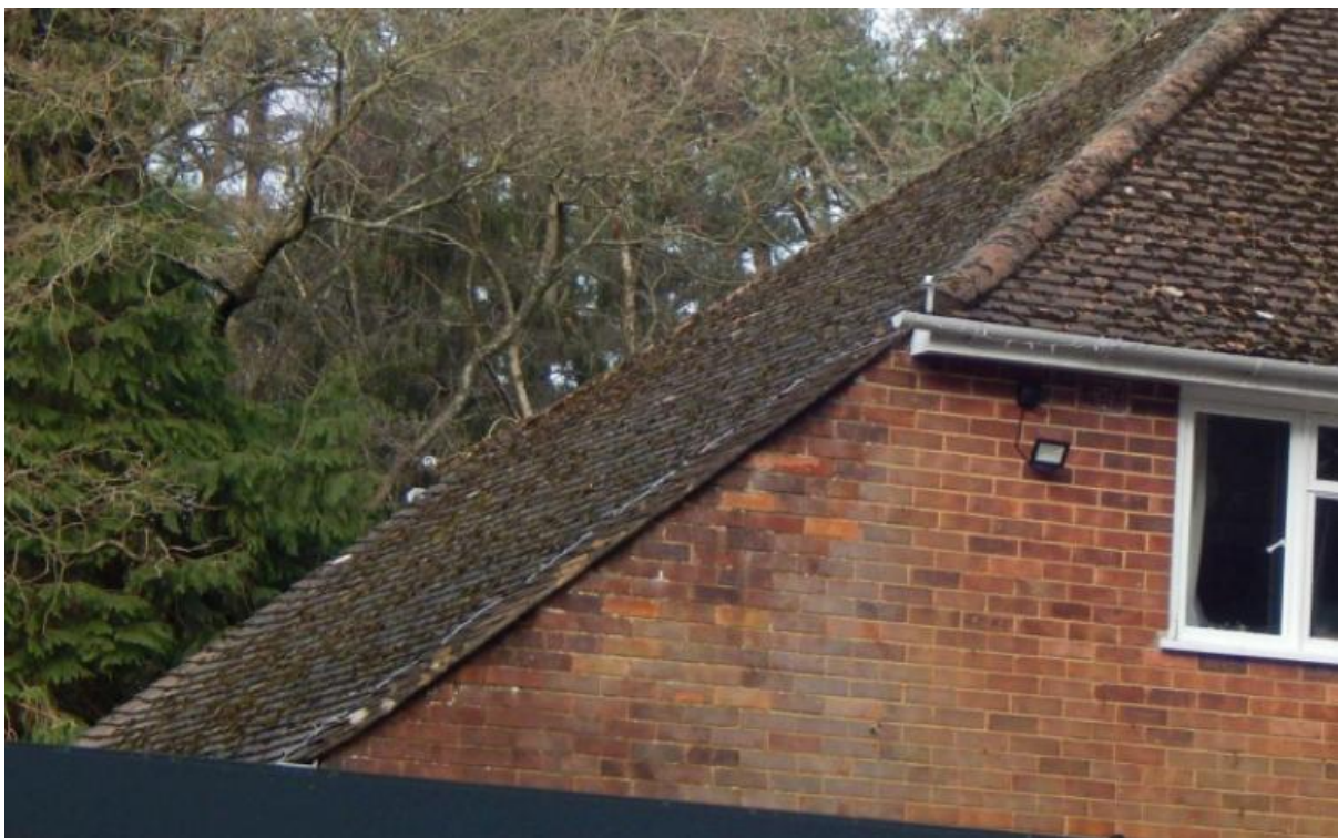
Image 6 – West facing elevation of the property
