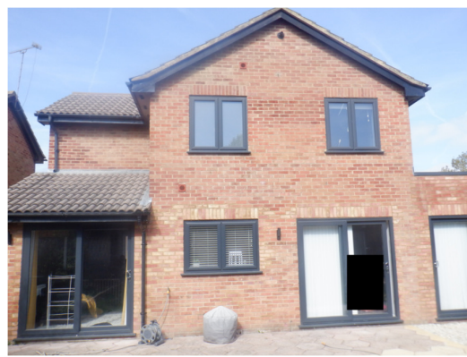
Photograph 2. Rear of property viewed from east.
