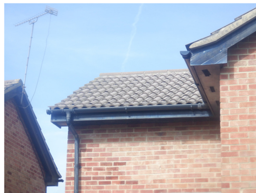
Photograph 4. Intact mortar along the ridge and gable (rear elevation).
