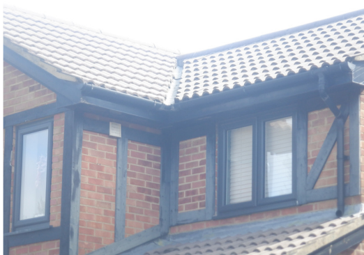
Photograph 3. Fully sealed roof tiles (front elevation).
