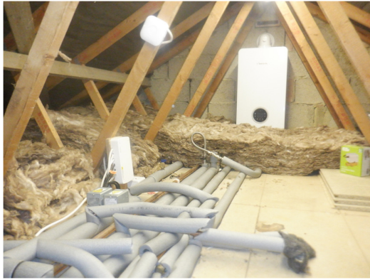
Photograph 10. Roof void of trussed construction
