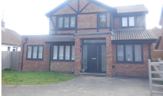
Photograph 1. Front of property viewed from west.
