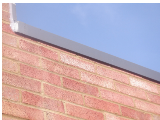
Photograph 8. Metal cap sealed to the brickwork (rear elevation).
