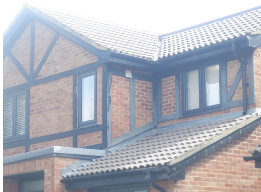
Photograph 6. Fully sealed lead flashing (front elevation).
