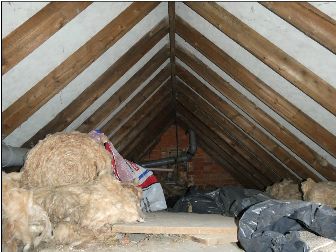
Figure 10. Example loft space of rear, single storey extension. Hillside House, Spencers Wood. 14.11.25
