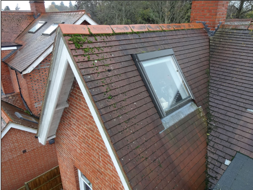
Figure 5. Example of sealed roof and ridge tiles. Hillside House, Spencers Wood. 14.11.25
