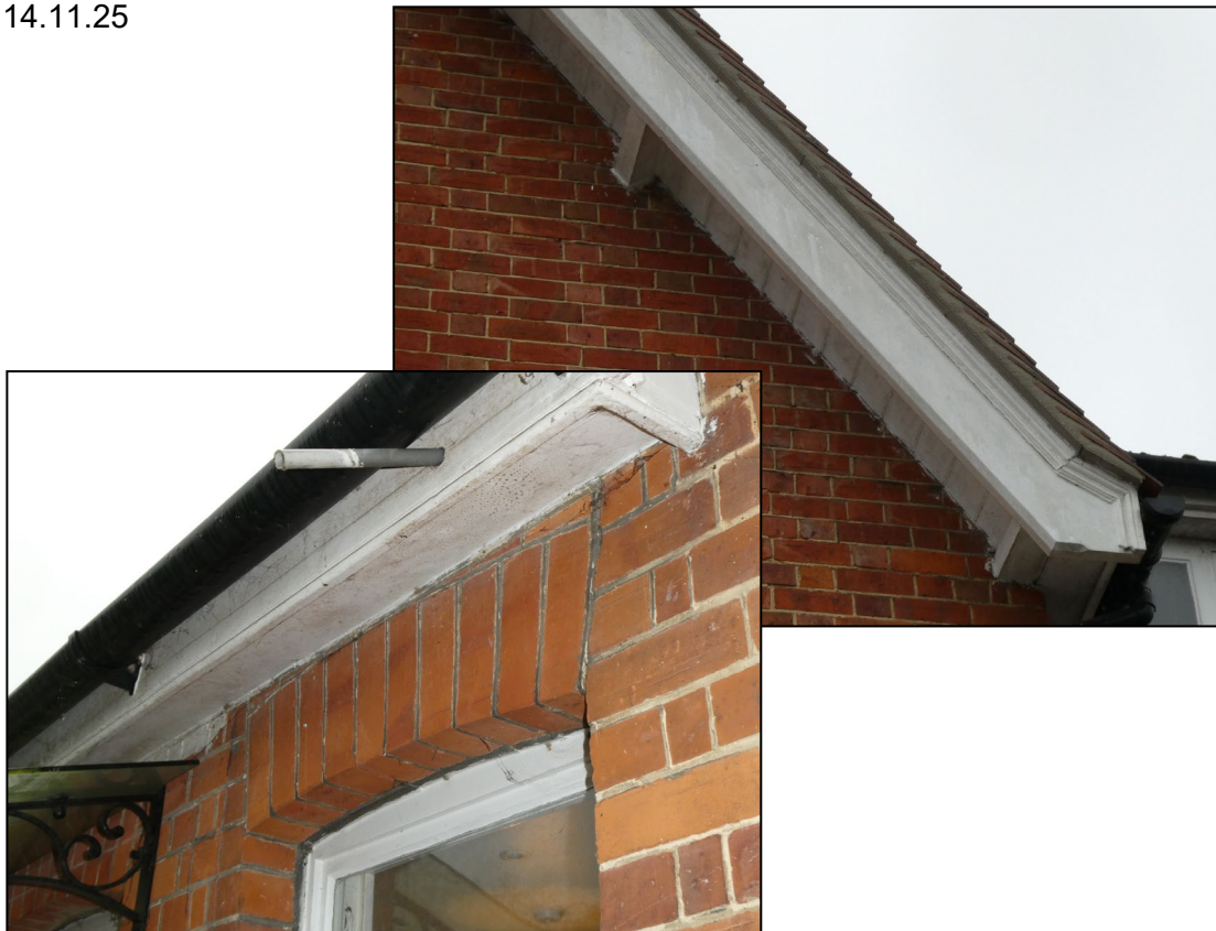
Figure 7. Example sealed soffits and fascias. Hillside House, Spencers Wood. 14.11.25
