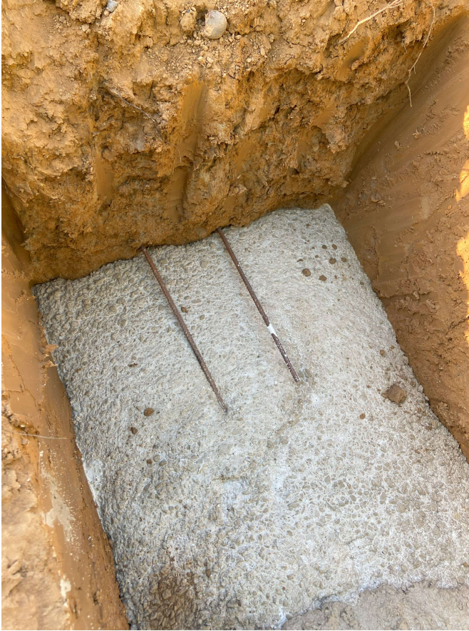
footing in progress (now complete)
