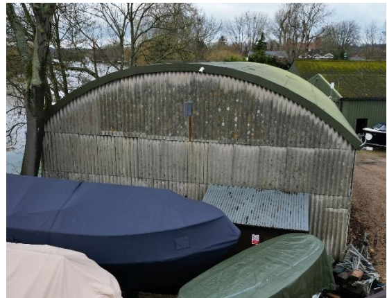
Current Rear of Shed 3
