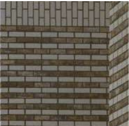
Contrasting brick band detailing
