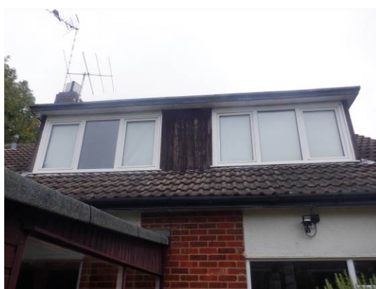
4. Vertical timber cladding on box dormers (rear elevation).
