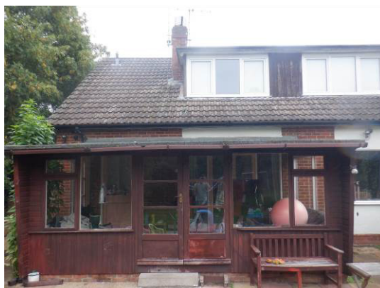
2. Rear of property viewed from south.
