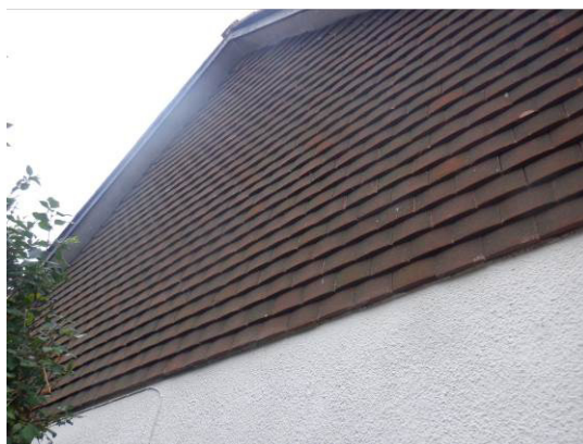
6. Hanging tiles on gable end (eastern elevation).
