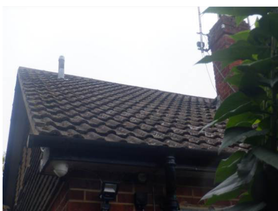
3. Interlocking roof tiles (rear elevation).
