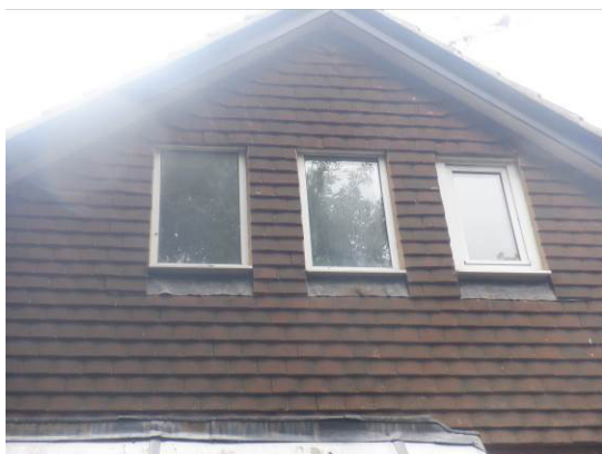
5. Hanging tiles on gable end (western elevation).
