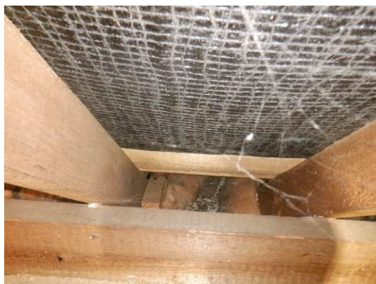
10. Fibreglass insulation in eaves (roof void).
