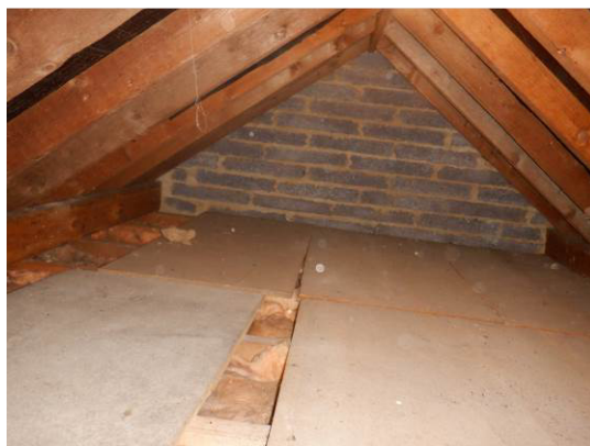
8. Roof void viewed from eastern end.
