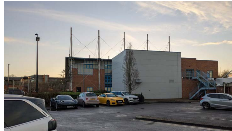
Photo 5 View 5 - Rear of existing club
