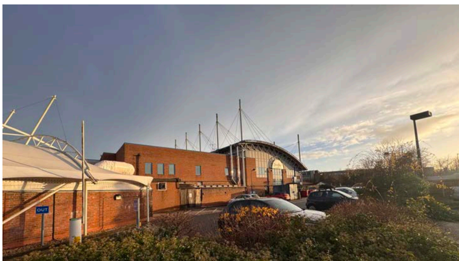
Photo 3 View 3 - Rear of existing club
