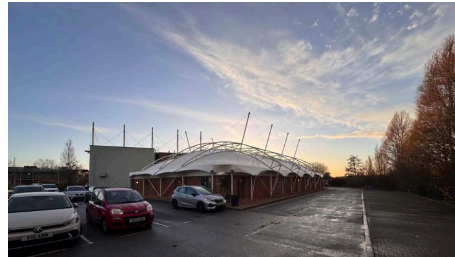
Photo 4 View 4 - Rear of existing pool
