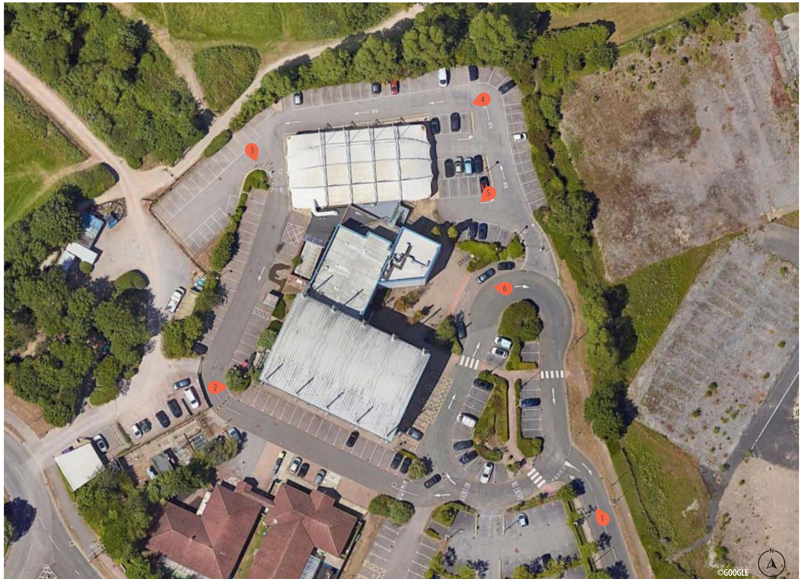
Fig. 3 Site Aerial Photograph
