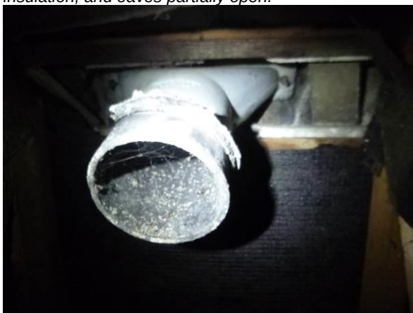
Photograph 13. Gap in felt around a pipe.
