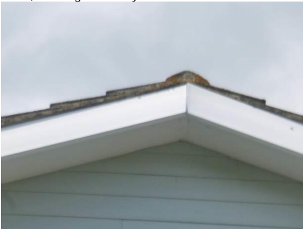
Photograph 5. Gap where the two soffit fascias joined on the rear roof elevation. Verge mortar intact.
