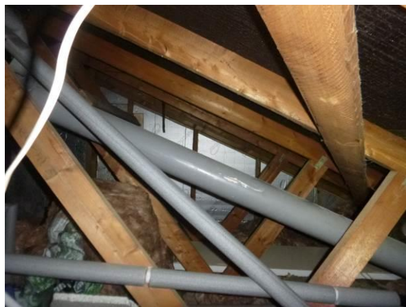
Photograph 14, The cluttered roof space.
