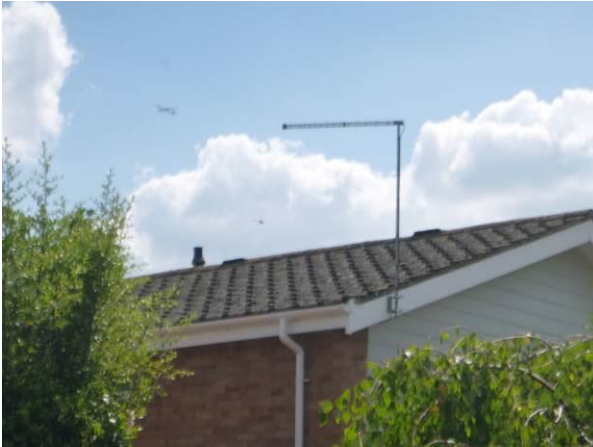
Photograph 3. Interlocking roof tiles in place and intact, and ridge tiles fully mortared.
