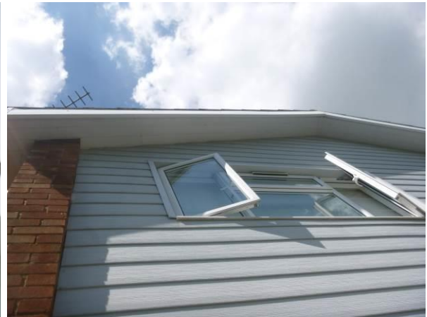
Photograph 6. Walls tightly clad with uPVC boards.
