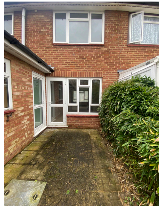
▲ EXISTING BUILDING - rear elevation
