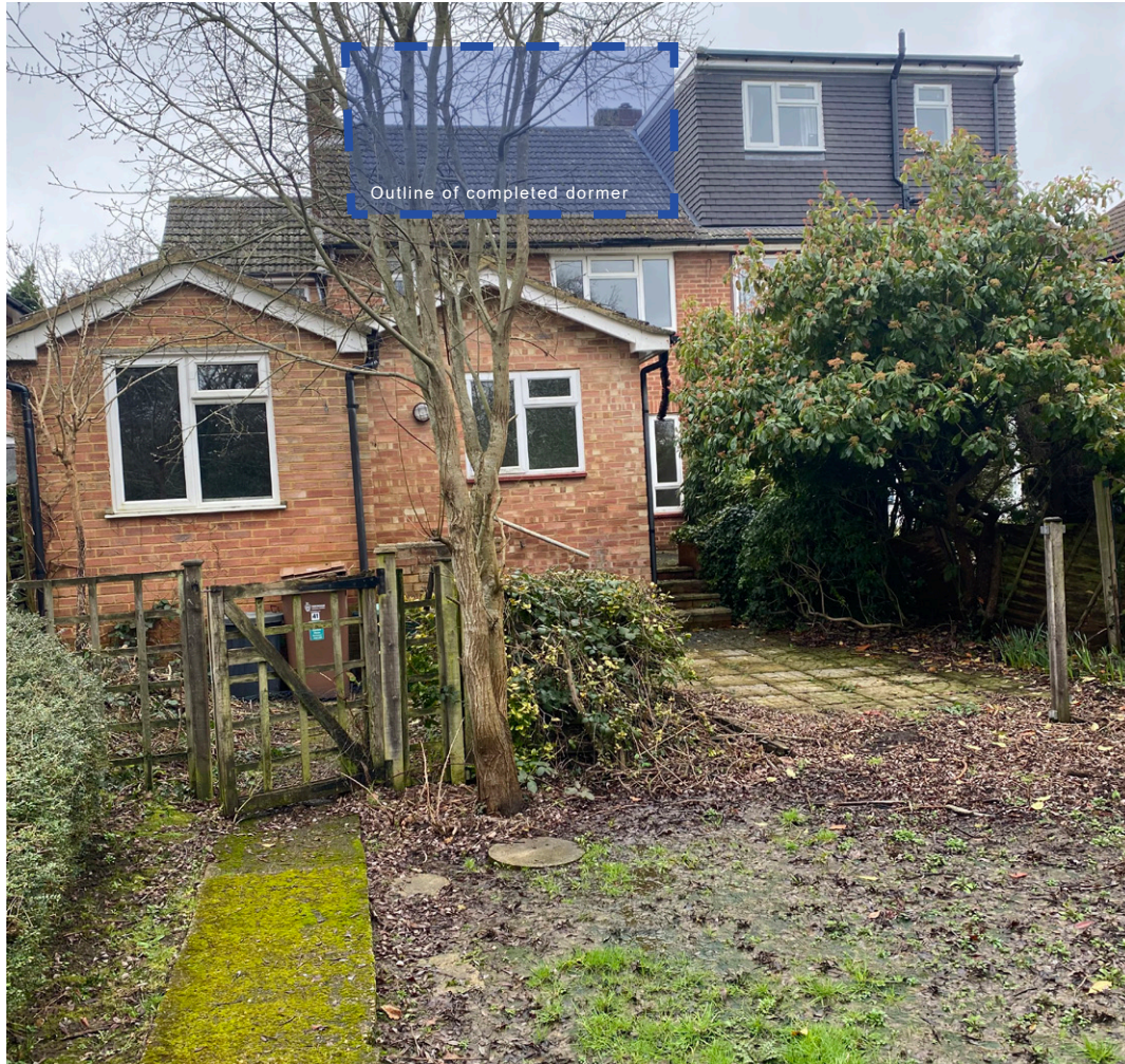
▲ EXISTING BUILDING - back garden and rear elevation
