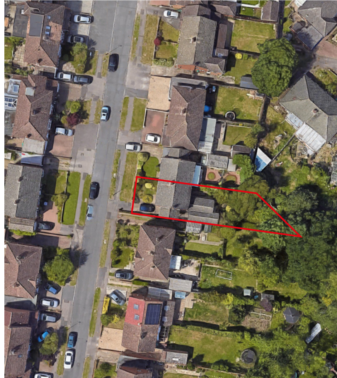
▲ AERIAL IMAGE - the site as existing
