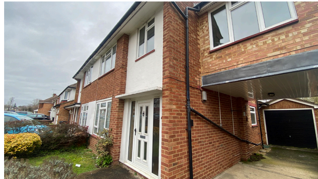
▲ EXISTING BUILDING - front entrance & elevation
