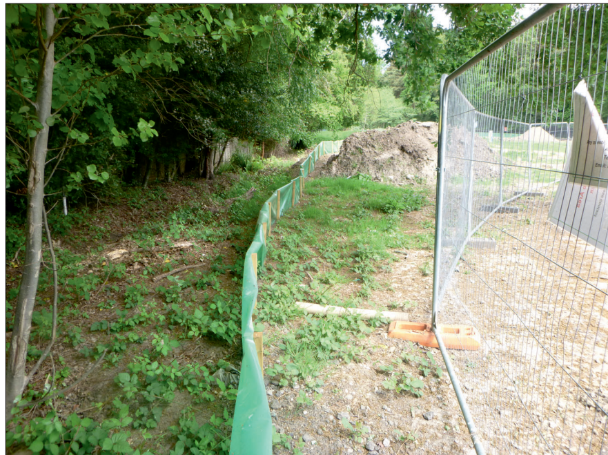
Photograph 3: Showing the reptile proof fencing and Heras fencing, with retained habitat to the left.
