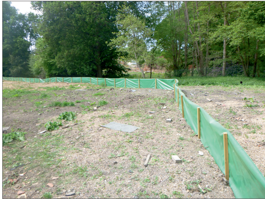
Photograph 1: Showing the reptile proof fencing, separating the 'construction zone' from the retained areas.
