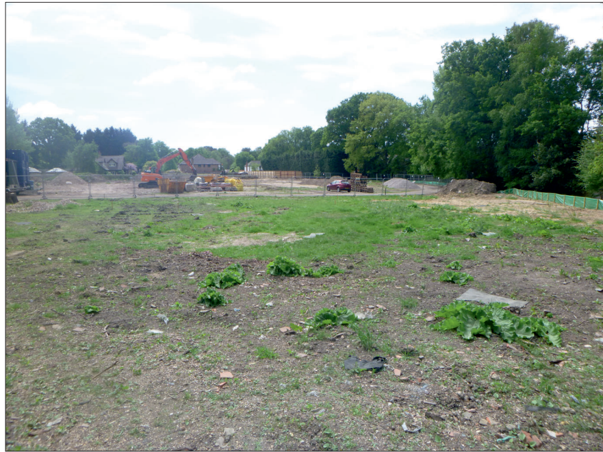
Photograph 2: Showing the 'construction zone' where the artificial refugia were placed.
