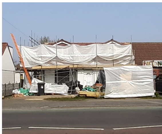
Figure 1 365 Wokingham Road. Image taken 23rd March 2026 showing front dormer extensions under construction.
