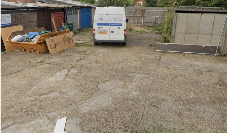
Current Site Ground Slab:
