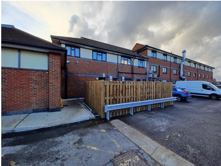
Figure 1: Photograph showing residential windows looking out across the application site.
