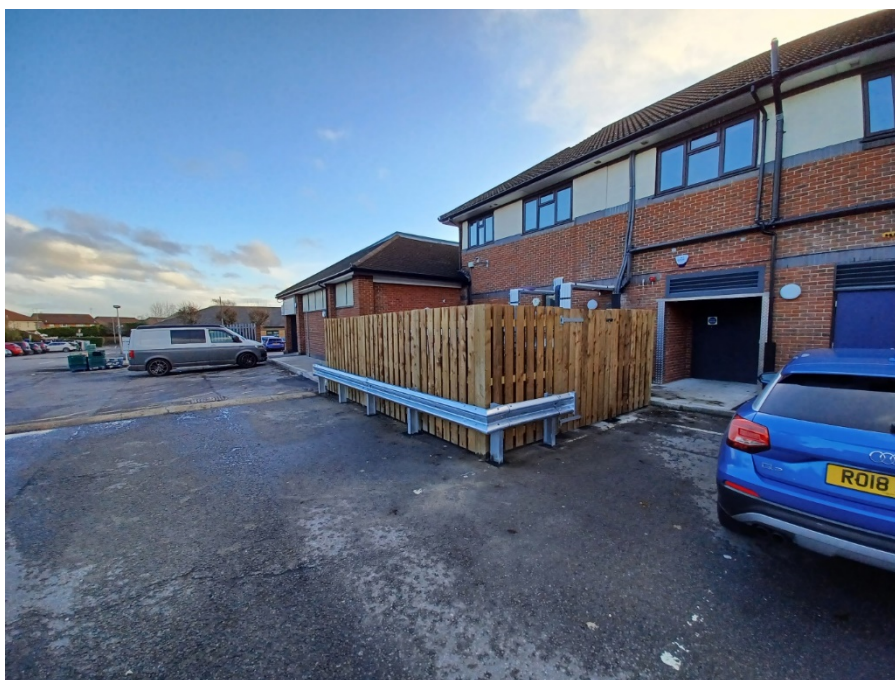
Figure 2: Photograph showing new access.
