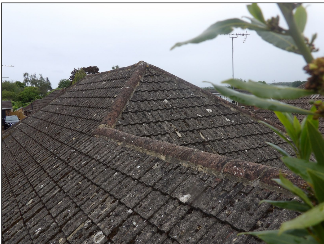
Figure 4. Example of sealed roof, ridge and hip tiles. 7 Paddock Heights, Twyford. 27.05.25
