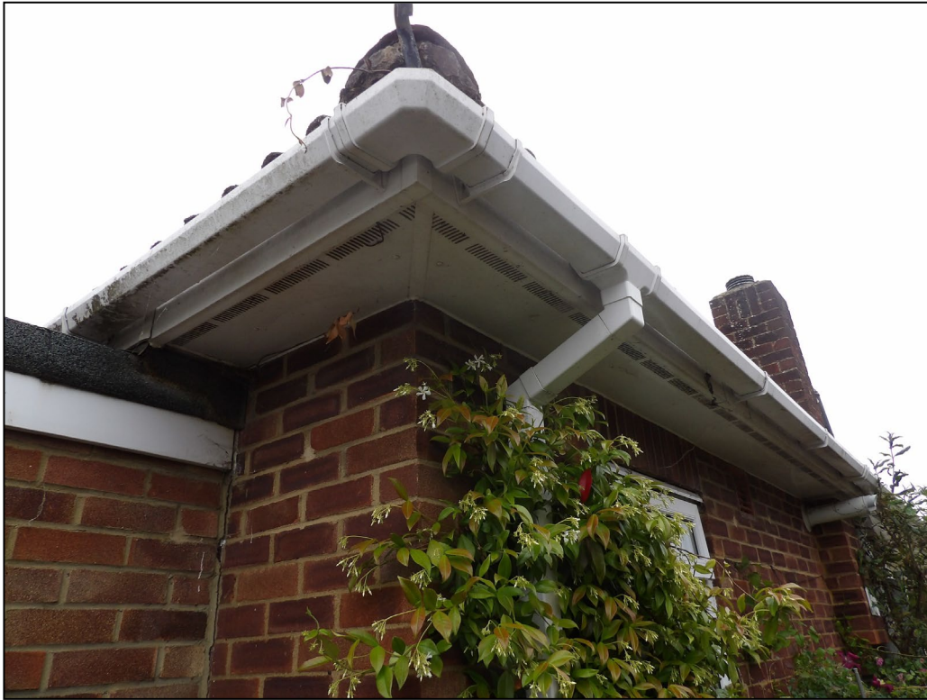
Figure 7. Example of soffits and fascias. 7 Paddock Heights, Twyford. 27.05.25
