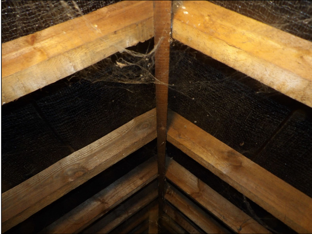
Figure 12. Example of bitumen lining. 7 Paddock Heights, Twyford. 27.05.25
