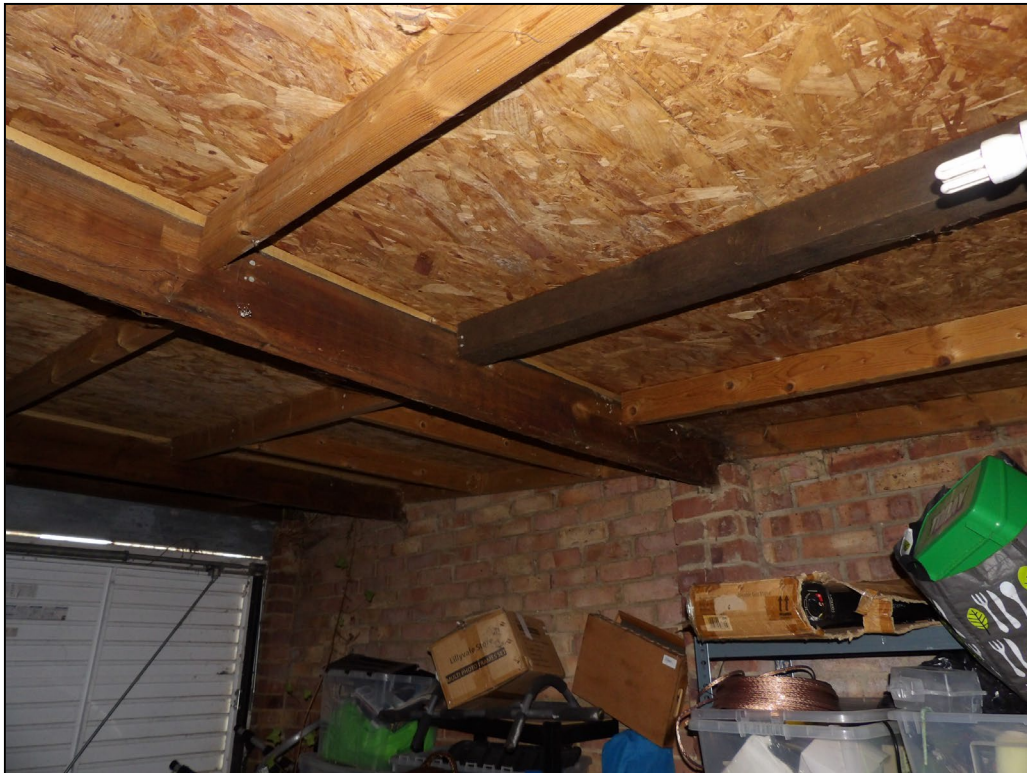
Figure 13. Internal view of garage roof. 7 Paddock Heights, Twyford. 27.05.25
