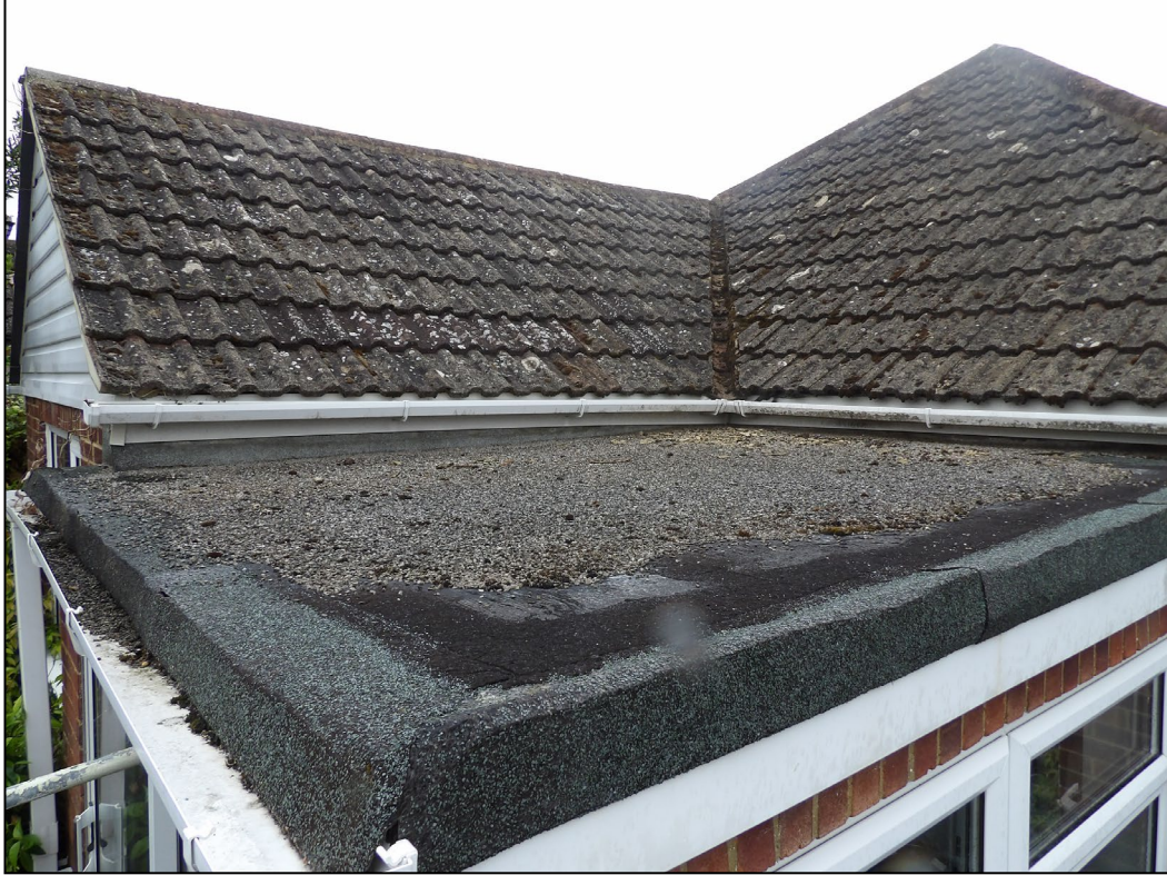
Figure 9. Bitumen covering on rear extension. 7 Paddock Heights, Twyford. 27.05.25
