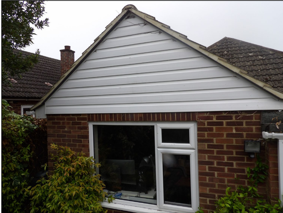
Figure 5. Example of sealed verge. 7 Paddock Heights, Twyford. 27.05.25
