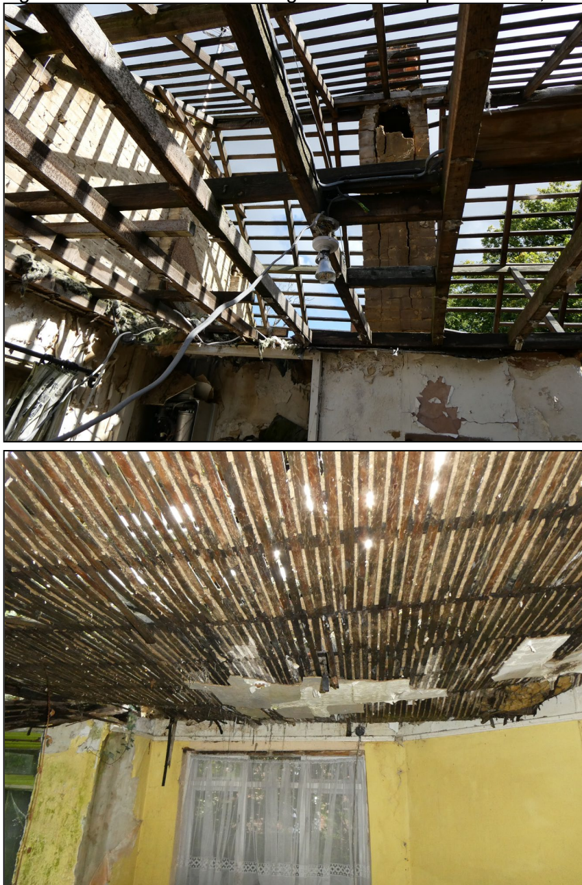
Figure 6. Internal view of building. 247 Finchampstead Road, Wokingham. 03.09.25
