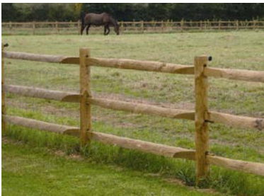
Heavy post & 3 rail fence
