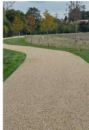
Bitumen bound gravel path
