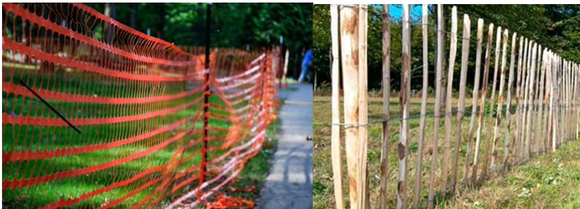
Figure C3 Tree protection fencing specification (Orange Weldmesh or Chestnut Pail)
