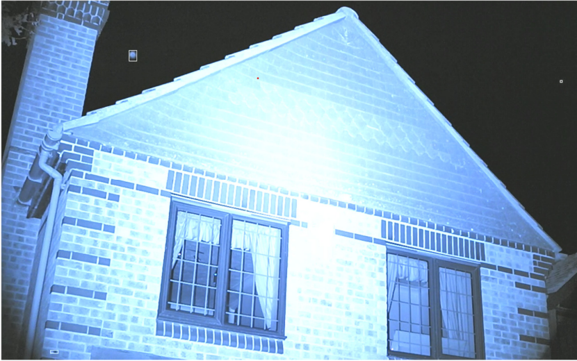
Sionyx Aurora Pro at Survey Location 1 on 30 th July 2024.
