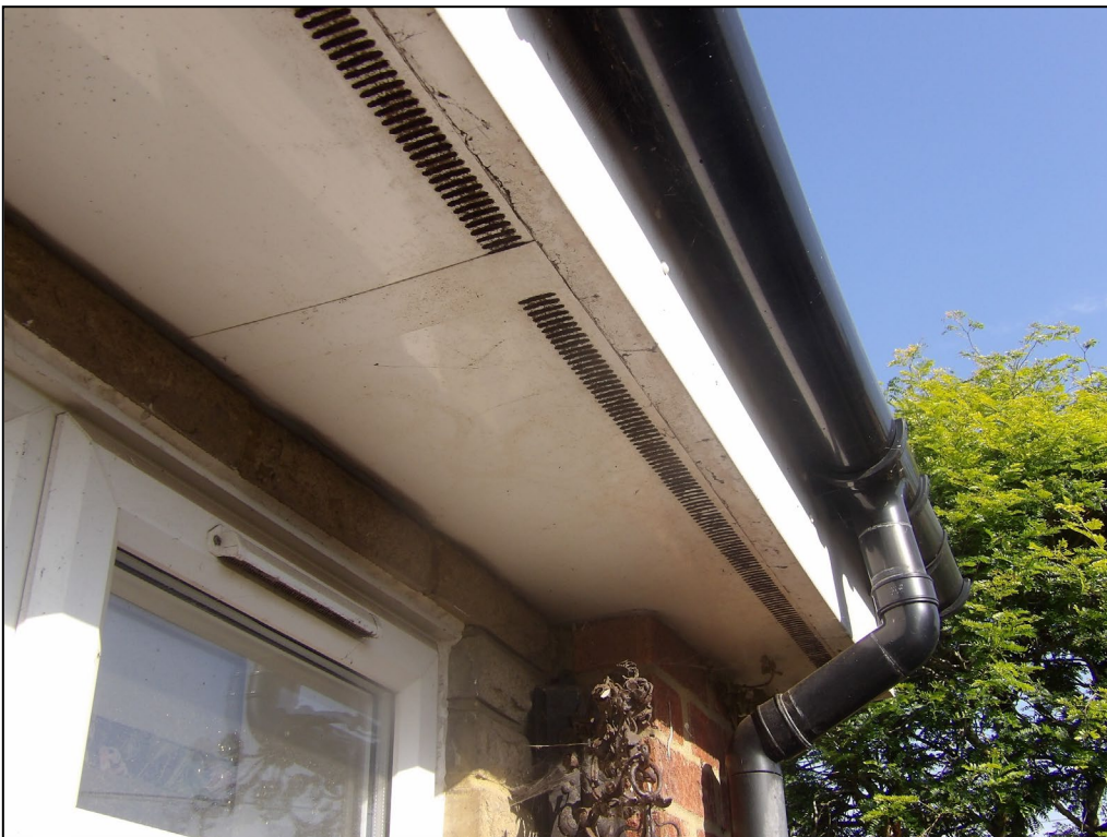
Figure 6. Example soffits and fascias. Greystones, 16 Aggisters Lane, Wokingham. 12.08.25
