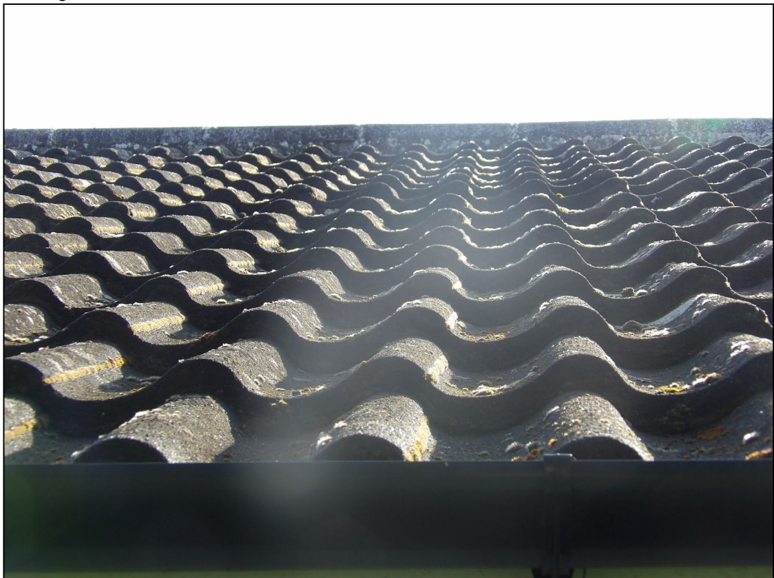
Figure 4. Example of sealed roof and ridge tiles. Greystones, 16 Aggisters Lane, Wokingham. 12.08.25
