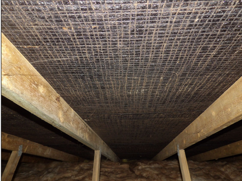
Figure 11. Example bitumen felt lining to tiles. Greystones, 16 Aggisters Lane, Wokingham. 12.08.25
