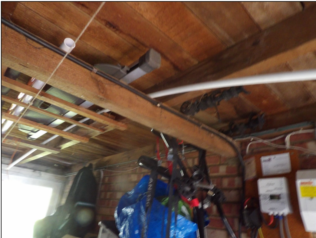
Figure 12. Interior view of garage and roof. Greystones, 16 Aggisters Lane, Wokingham. 12.08.25
