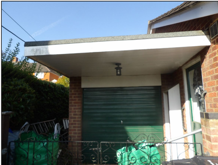
Figure 7. Garage. Greystones, 16 Aggisters Lane, Wokingham. 12.08.25
