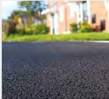
Macadam surfacing with flat top concrete edging
