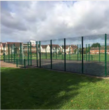
Green weld mesh fencing around MUGA Dimensions: 3000mm height above ground Example shown: Mant Leisure
