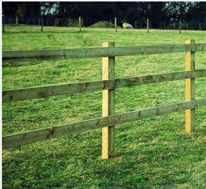
3 rail, square post and rail fencing
