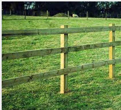
3 rail, square post and rail fencing
