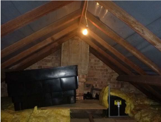
Photograph 8. Cobwebbed ridge (roof void).
