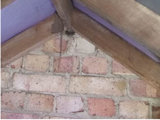
Photograph 12. Cobwebbed brickwork party wall (roof void).
