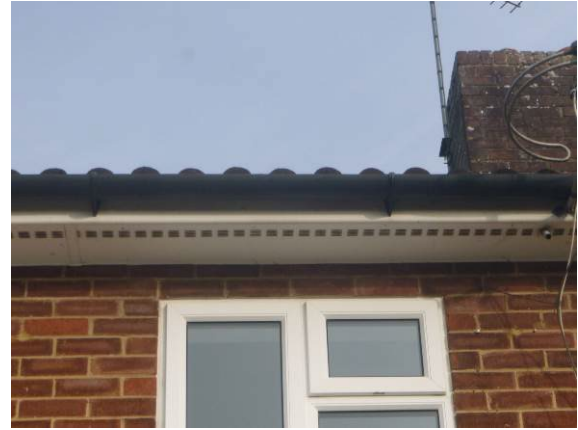
Photograph 6. Intact sealant present along uPVC soffit (rear elevation).
