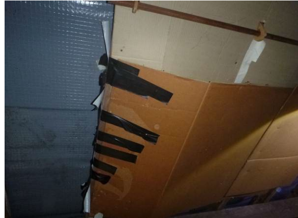
Photograph 9. Intact plastic backed hessian roofing felt (roof void).
