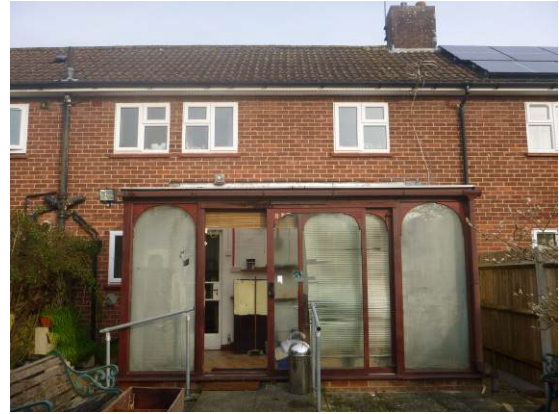
Photograph 2. Rear of the property, viewed from the south.
