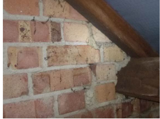
Photograph 13. Brickwork party wall tight to rafters (roof void).
