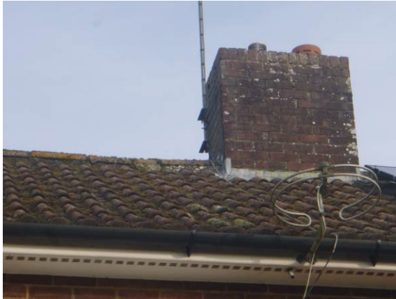
Photograph 5. Tight lead flashing around chimney on the party end of the roof (rear elevation).
