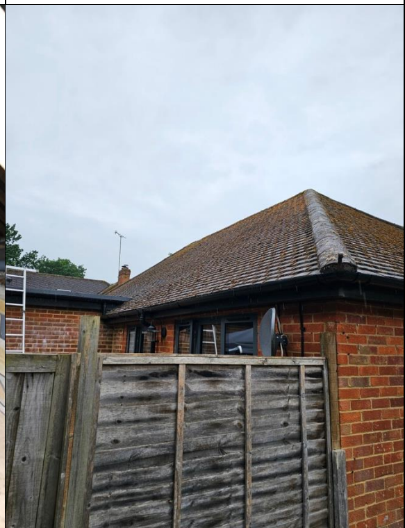
Photograph 4: No gaps under roof tiles.
