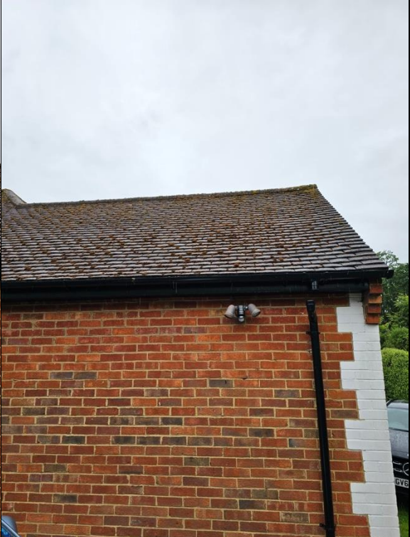
Photograph 8: No visible gaps under roof tiles.
