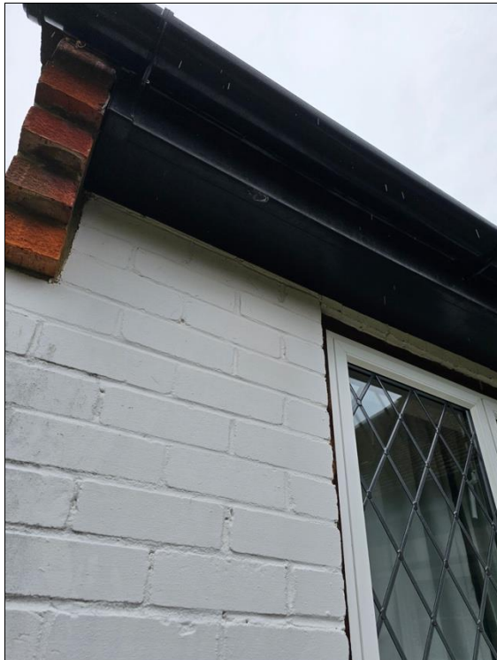
Photograph 1: New uPVC soffits.
