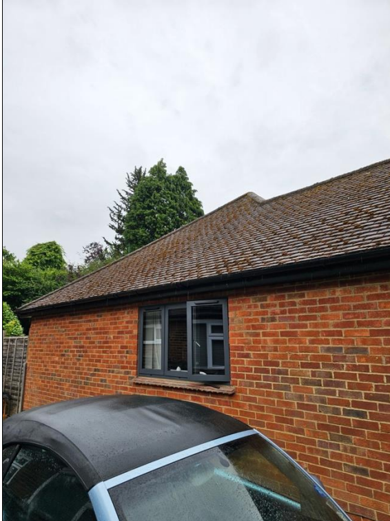
Photograph 7: No visible gaps under roof tiles.
